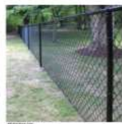
10 Chain Link Fence July 2016
