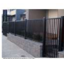
9 3-FT High CMU Wall with 3-FT High Taper Steel Fencing July 2016
