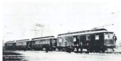
The Electric Railway and Interurban Depots
