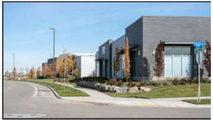
EXISTING SINGLE-STORY SHOPS
