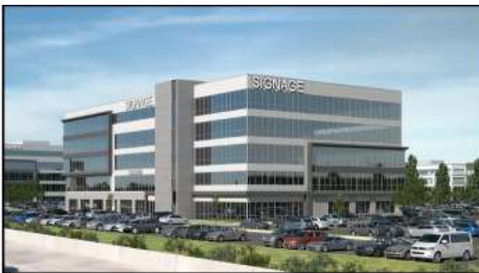
LASALLE BUILDING (under constr)
