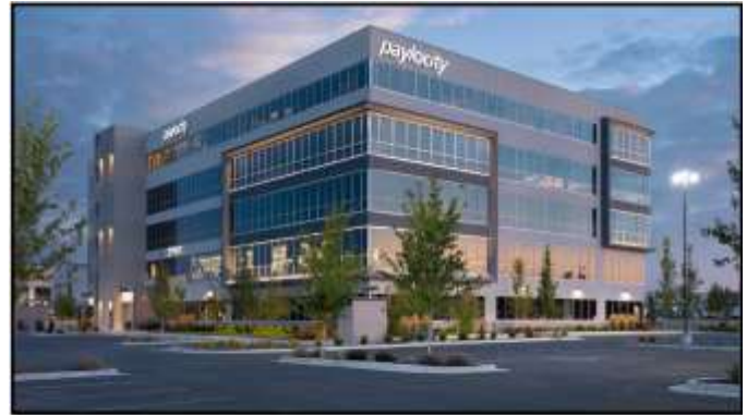
PAYLOCITY BUILDING (complete)
