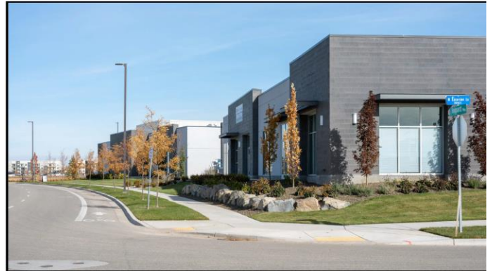
EXISTING SINGLE-STORY SHOPS
