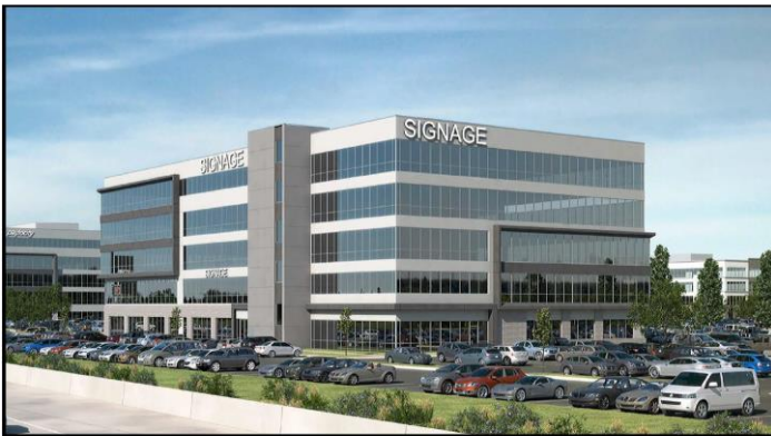
LASALLE BUILDING (under constr)
