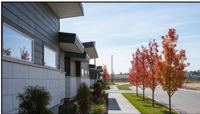
THE LOFTS at TEN MILE ( garages )
