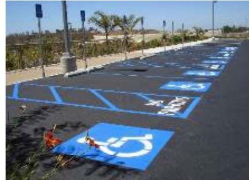
Example: ADA compliant striping (surface lot)
