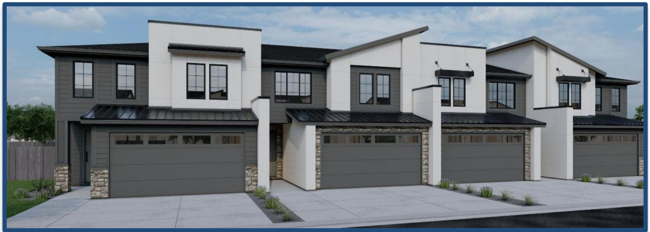
Paired Street Accessed Homes
