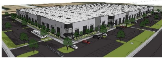
SOUTH EAST AERIAL
