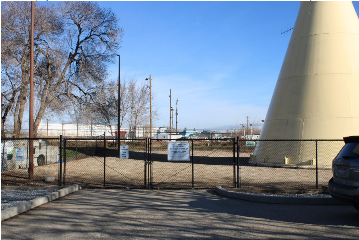
Photo 5 of 10. ID_AdaCounty_Meridian Water Tower 005 Meridian Water Tower, looking north to access gates. Photo by Barbara Perry Bauer, March, 2026.
