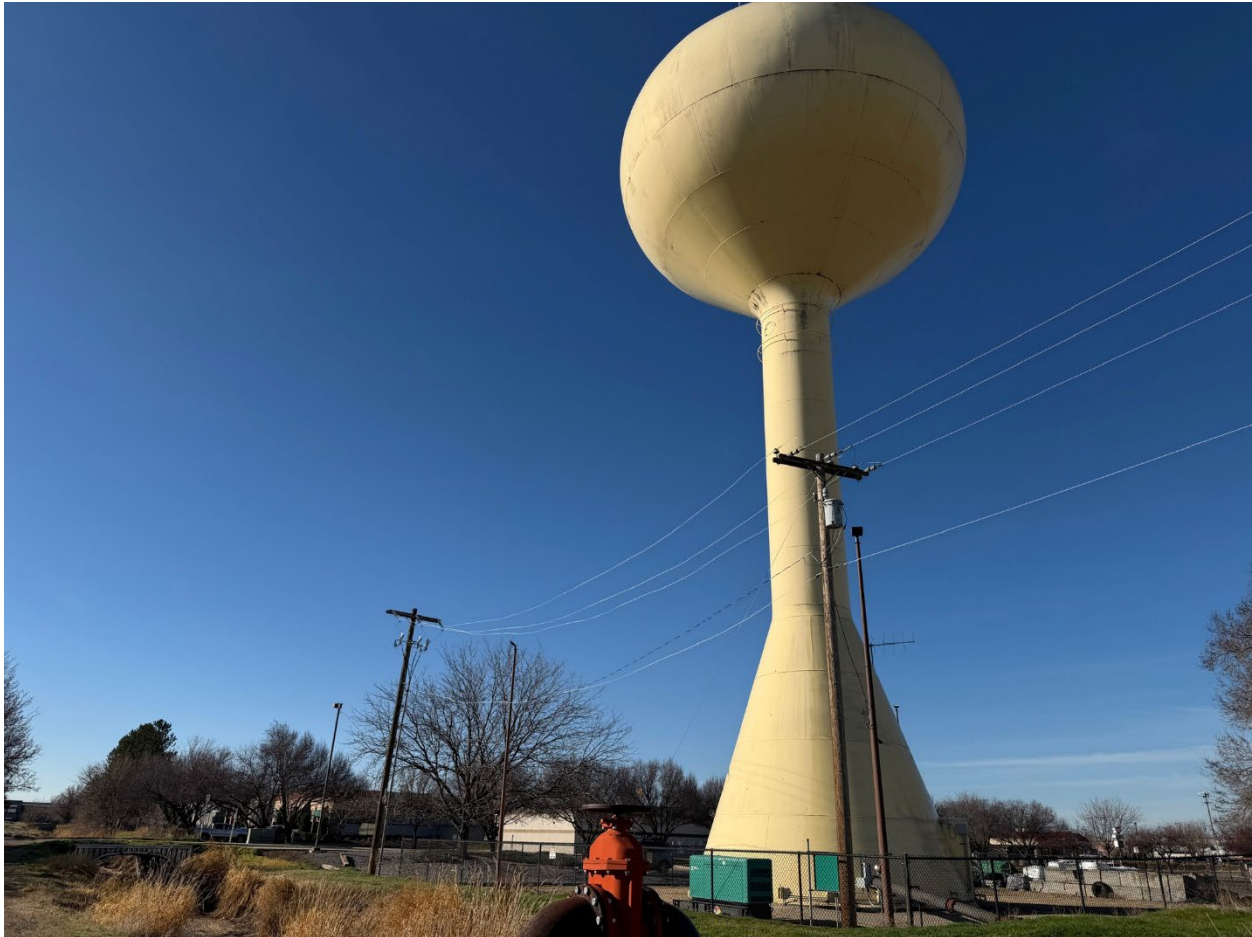
Photo 3 of 10. ID_AdaCounty_Meridian Water Tower 003 Meridian Water Tower, facing southwest. Photo by Jeffery Holley, March, 2026.
