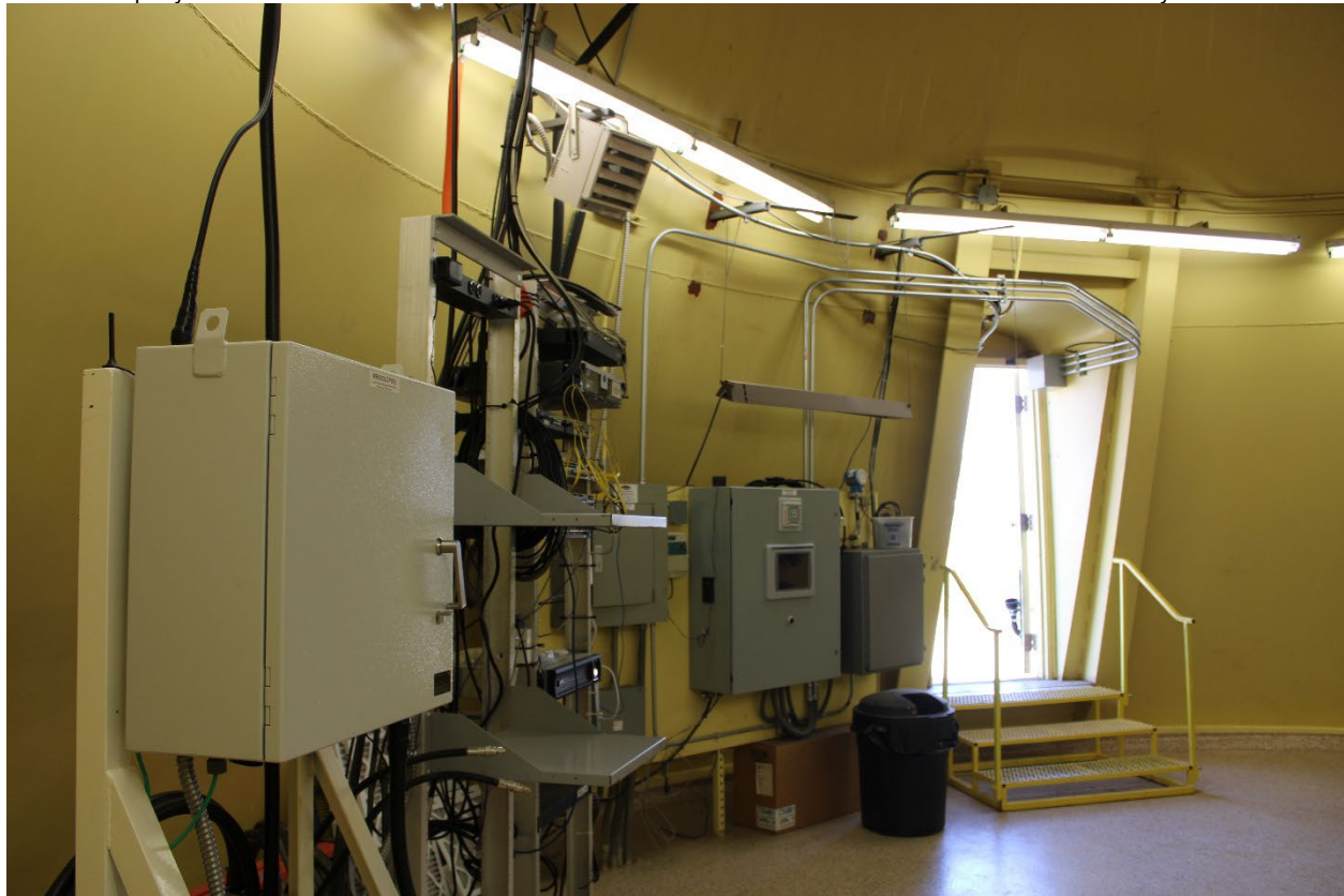
Photo 9 of 10. ID_AdaCounty_Meridian Water Tower 009 Meridian Water Tower, Interior. Camera facing north. Photo by Barbara Perry Bauer, March, 2026.
