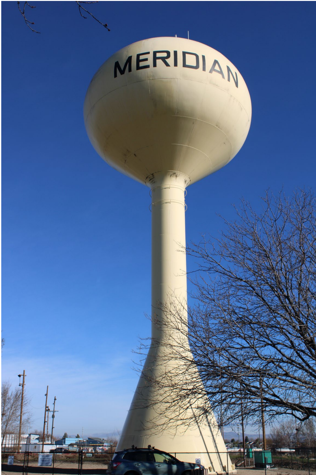
Photo 2 of 10. ID_AdaCounty_Meridian Water Tower 002 Meridian Water Tower, facing northeast. Photo by Barbara Perry Bauer, March, 2026.
