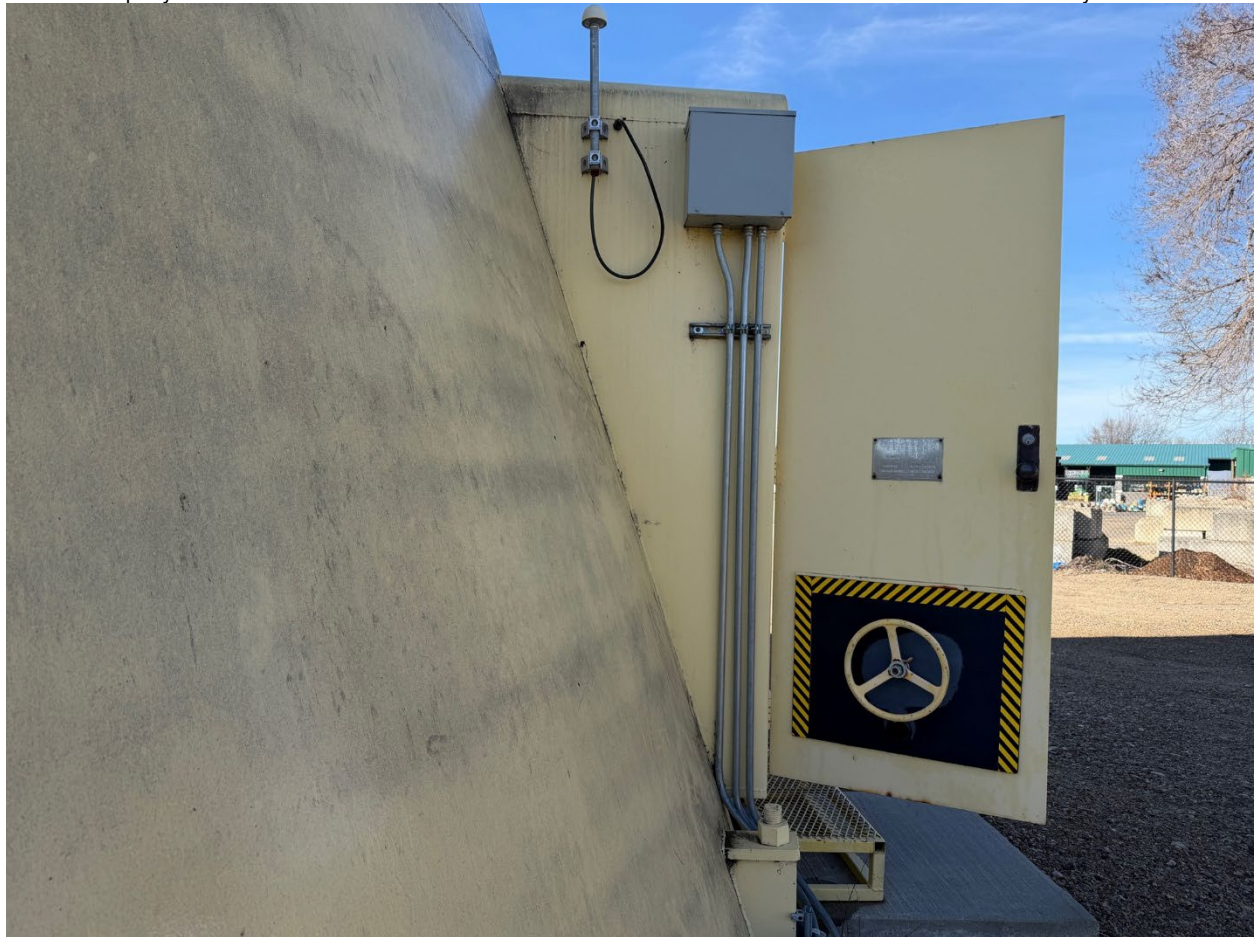
Photo 7 of 10. ID_AdaCounty_Meridian Water Tower 007 Meridian Water Tower, looking at entrance door. Camera facing west. Photo by Jeffery Holley, March, 2026.
