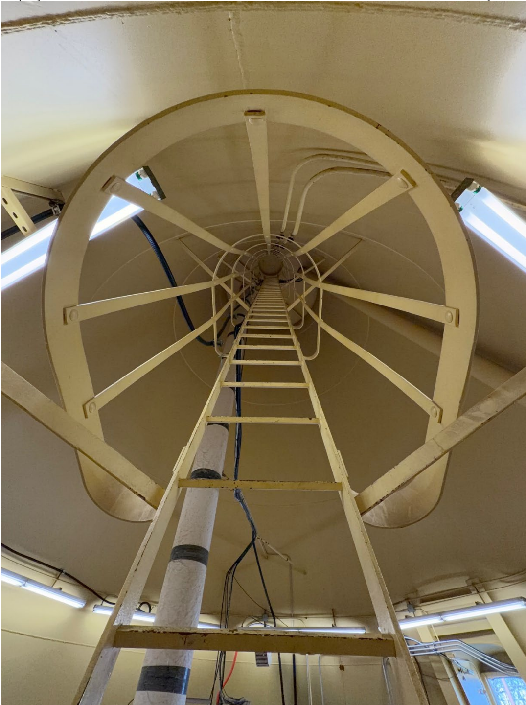
Photo 10 of 10. ID_AdaCounty_Meridian Water Tower 010 Meridian Water Tower, Interior view of access ladder. Camera facing west. Photo by Jeffery Holley, March, 2026.
