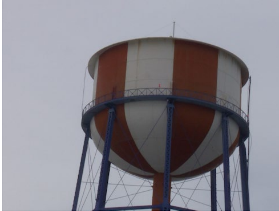
Idaho Falls Water Tower replaced 2026
