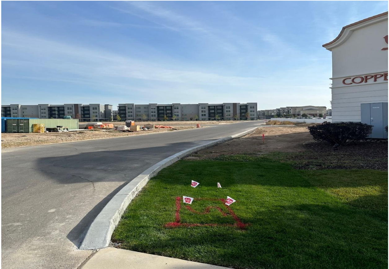
Access Road Entering the Development Complex North of Copper Canary
