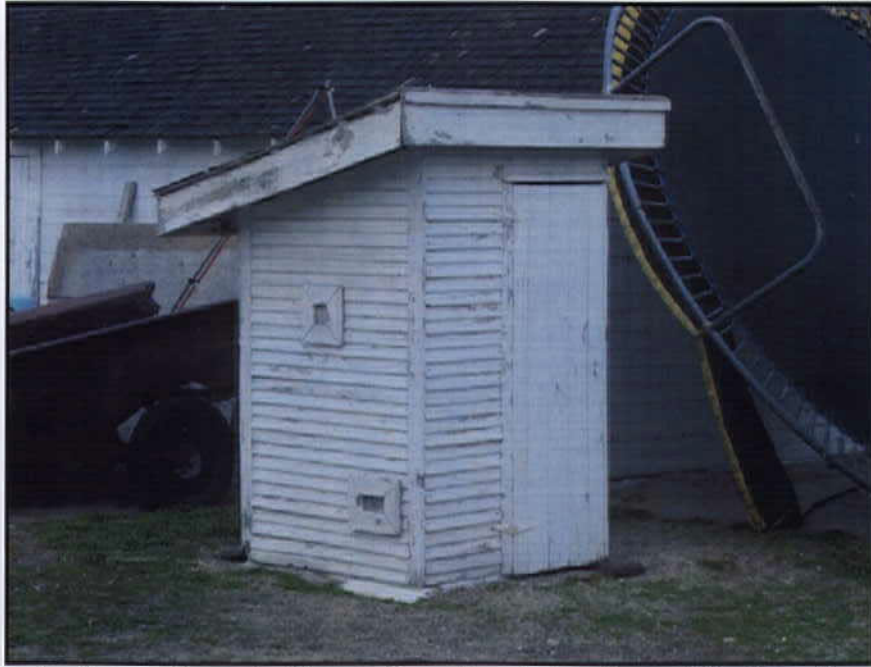
View looking northwest at the south and east elevations of No.13 outhouse.
