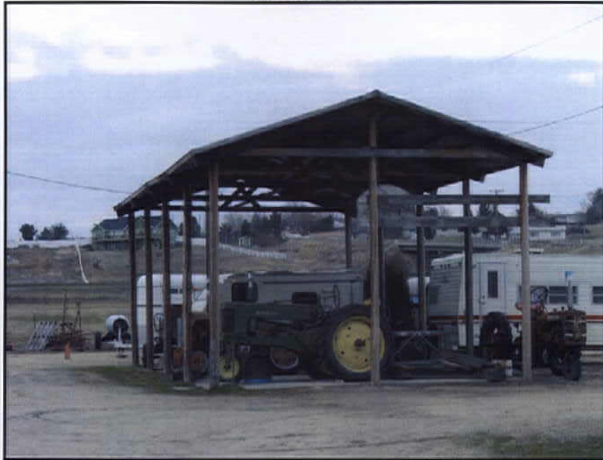
View looking southwest at the north and east elevations of No.11 wood shed.
