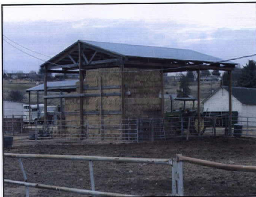
View looking southwest at the north and east elevations of No.10 pole shed.
