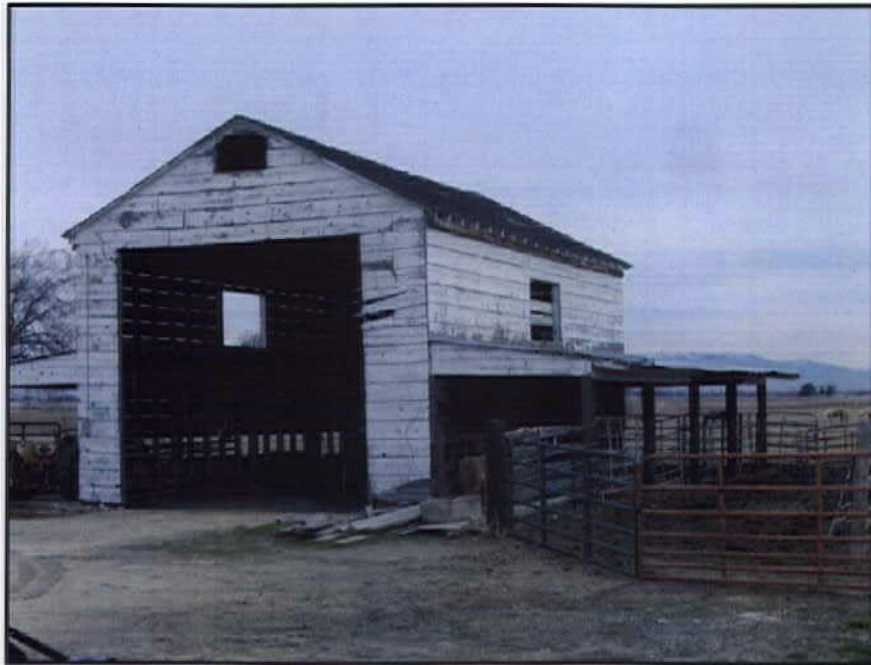
View looking northeast at the south and west elevations of No.14 feeder barn.
