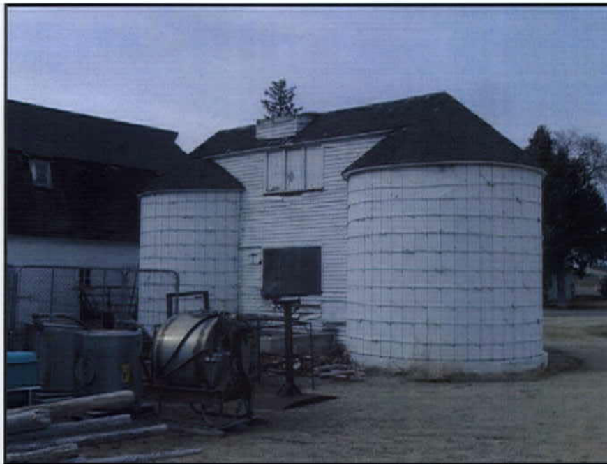
View looking southwest at the north and east elevations of No. 3 granary.
