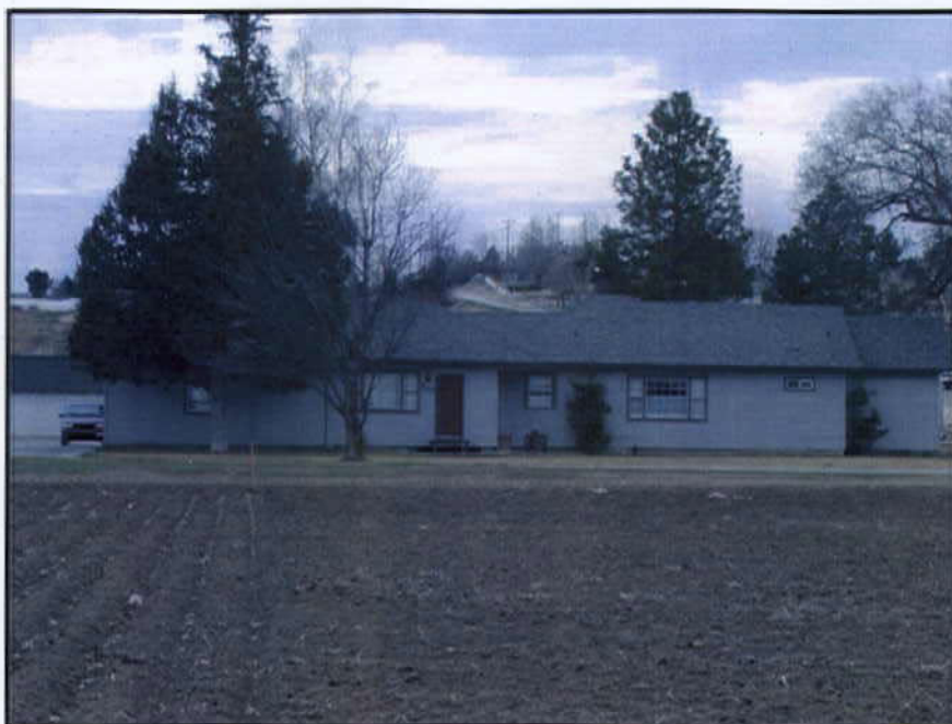
View looking south at the north elevation of No.1 house.
