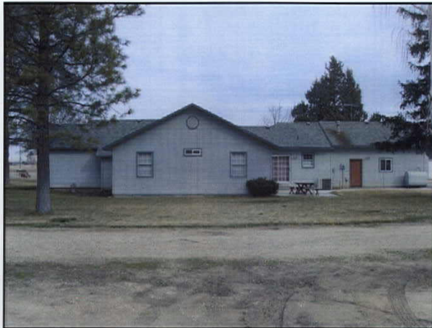
View looking north at the south elevation of No.1 house.
