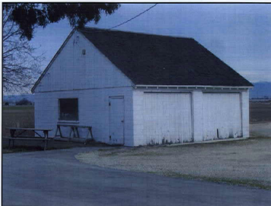
View looking northeast at the south and west elevation of No. 2 shop.
