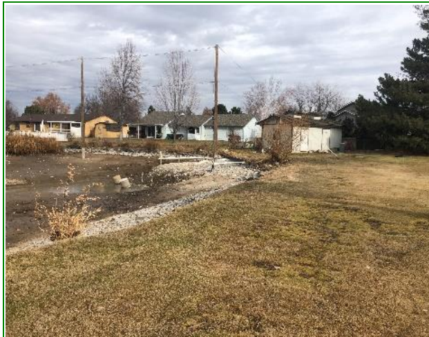
The pump station house adjacent to the small portion of the main irrigation lake that has been isolated to provide a winter reservoir for irrigation water needs.
