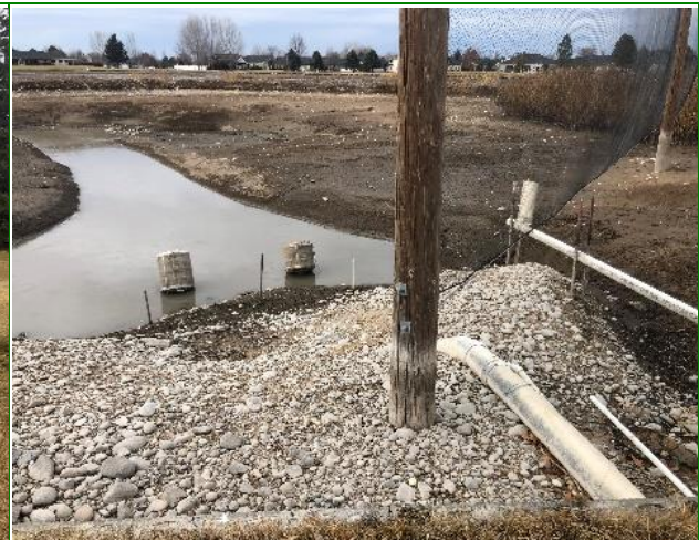
The intake pipe from the isolated reservoir of the main lake system.
