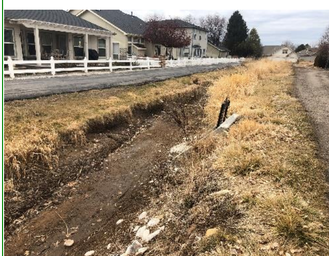
Water is supplied to the course by way of a canal system called the “Eight Mile Lateral,” of which this feeding ditch is the point at which water is allowed to flow into the main irrigation lake.
