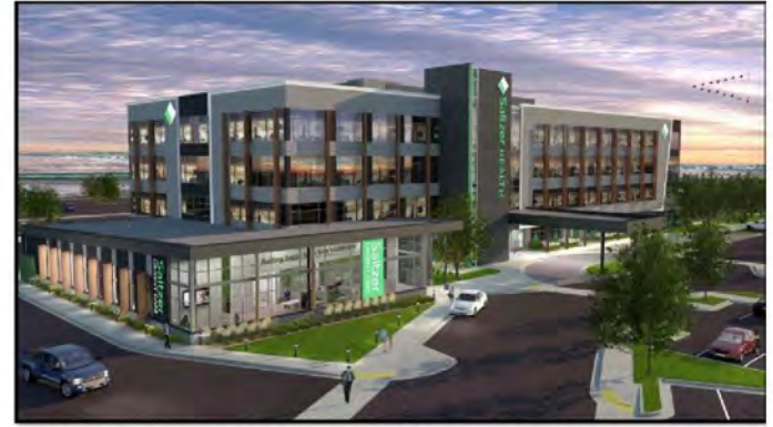
SALTZER MEDICAL (under constr)
