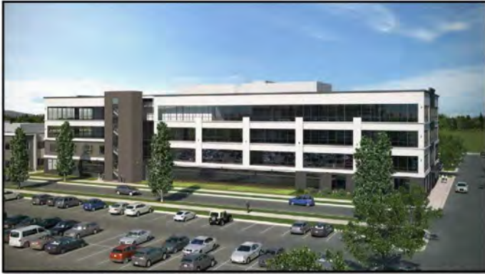
AMERIBEN PHASE II (under constr)
