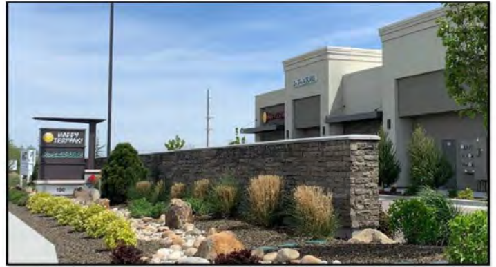
EXISTING RESTAURANT/SHOPS ( rear )
