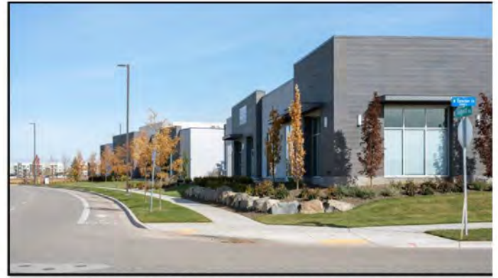
EXISTING SINGLE-STORY SHOPS
