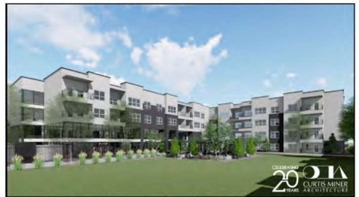
THE FLATS at TEN MILE ( under constr )
