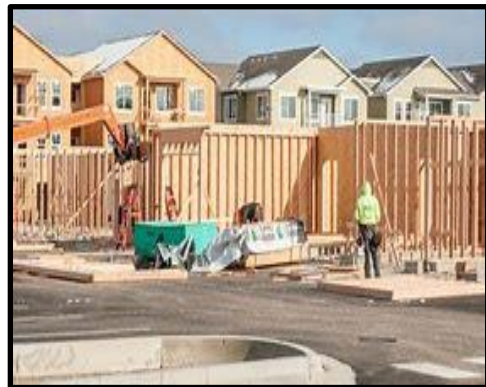
Meridian Housing - Single Family (Construction)
