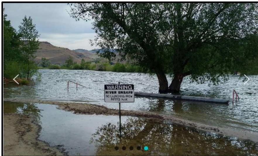
Flooding Along Boise River
