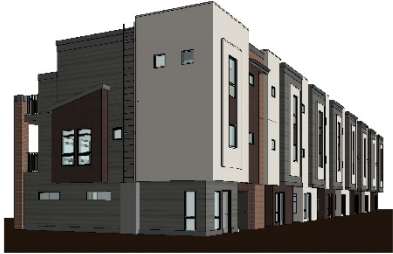
3 WILSON LN LOOKING NW
