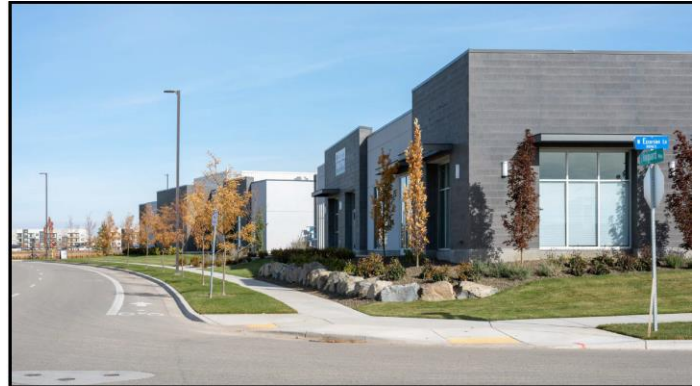
EXISTING SINGLE-STORY SHOPS
