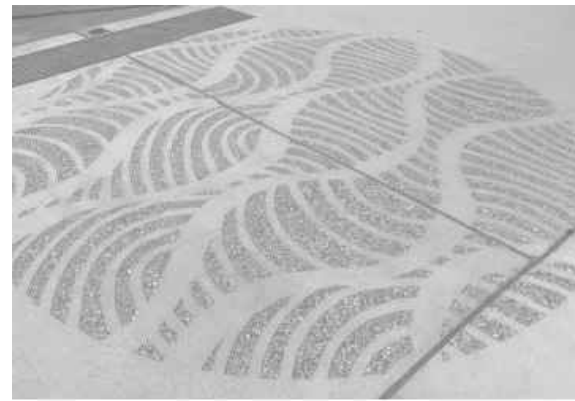
SANDBLASTED CONCRETE EXAMPLE
