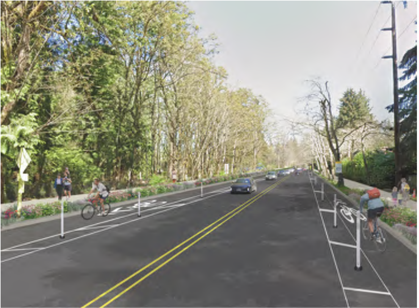
Figure 1: Separated Bike Lane
