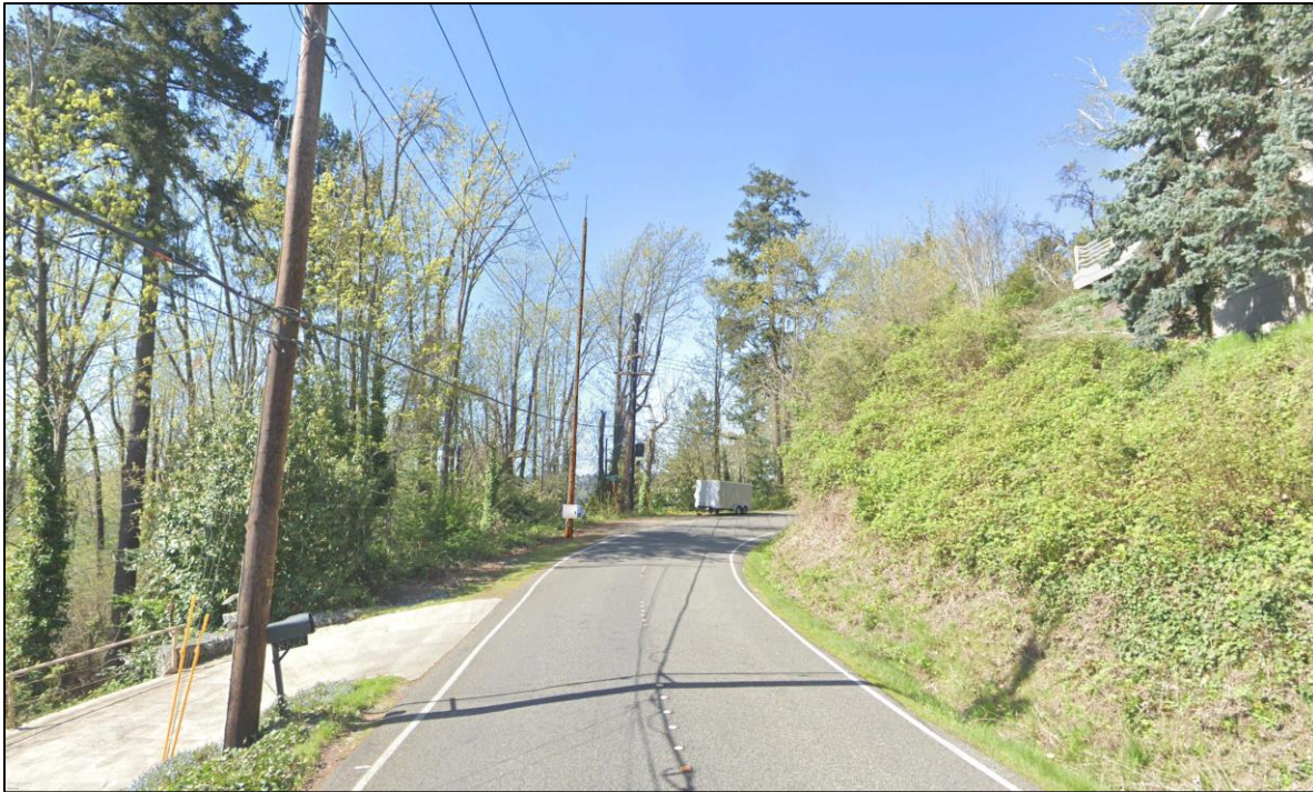
New 50' City-owned pole
