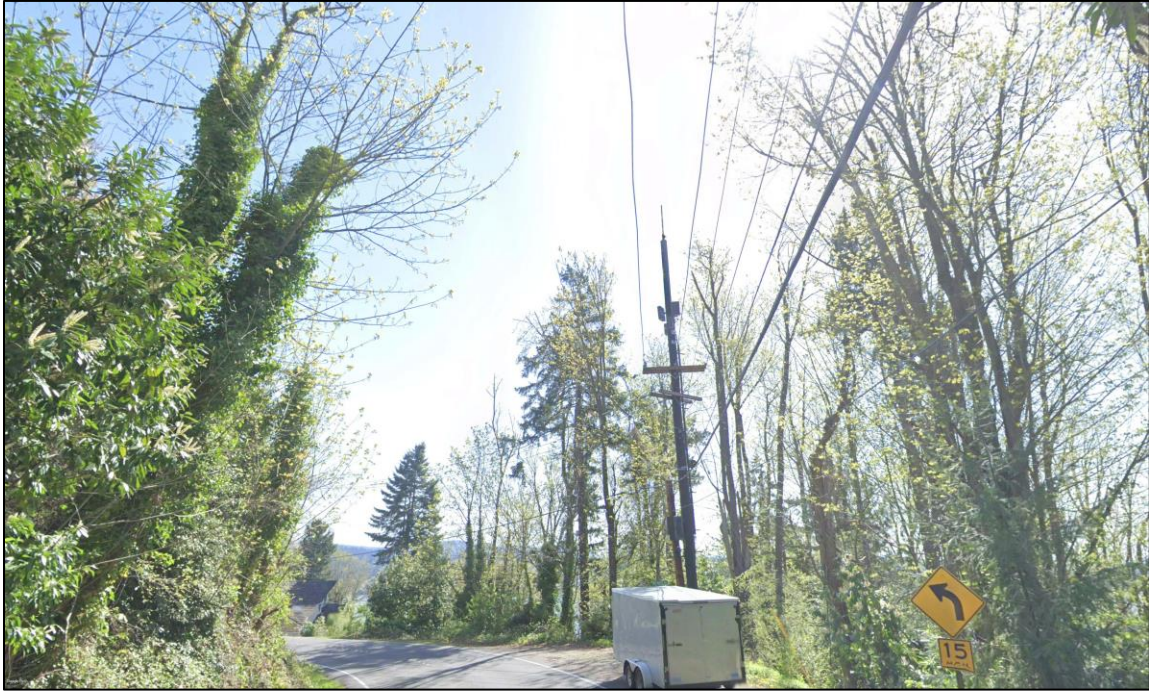
PSE-owned pole, replaced with 50' pole
