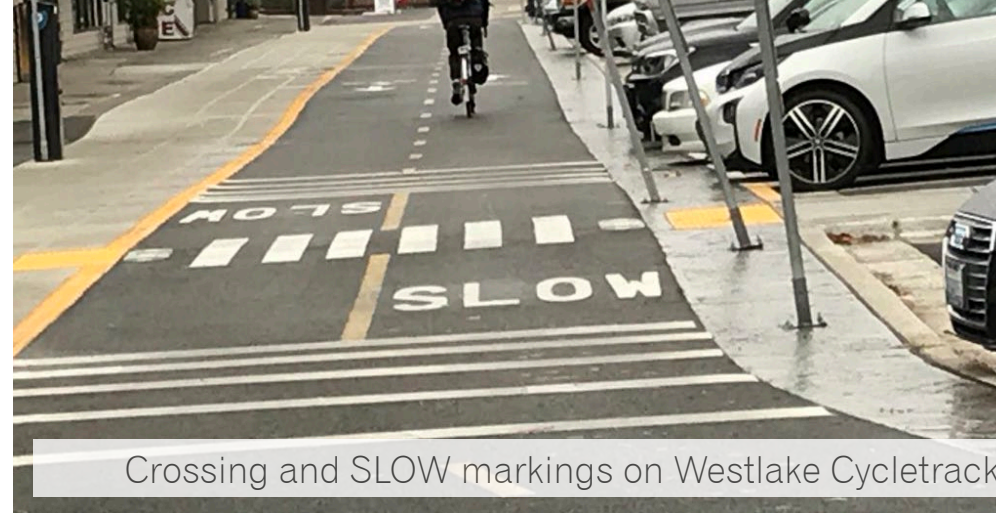
Yield line markings and signage on Elliott Bay Trail
