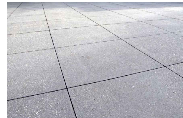
SAWCUT CONCRETE EXAMPLE
