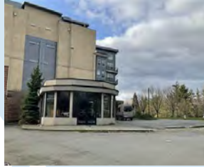
Tully's Building (Decommissioned)
