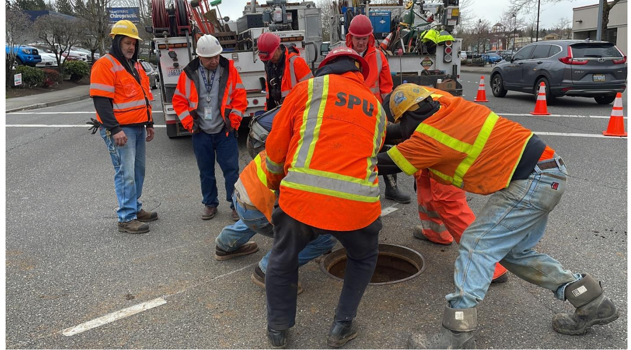
Crews manually turning the valve using a t-wrench attached to the top valve gear
