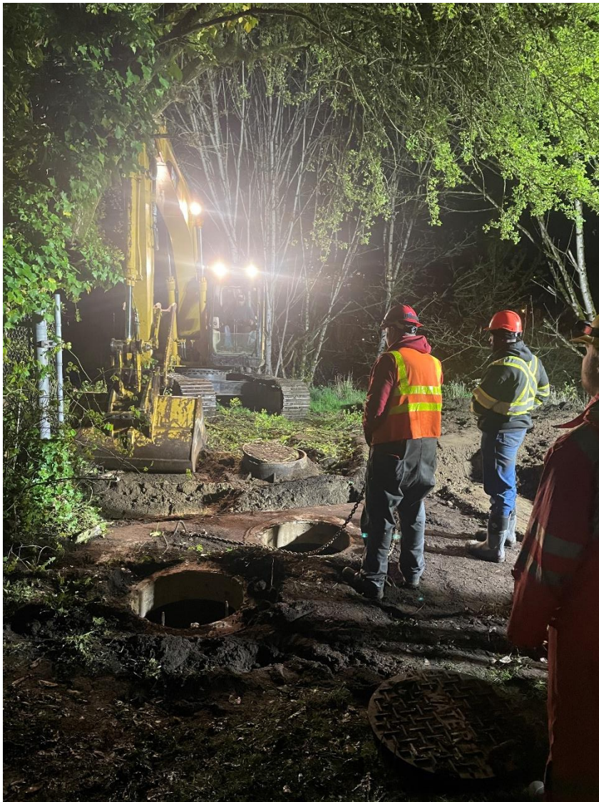
Valve vault before excavation
