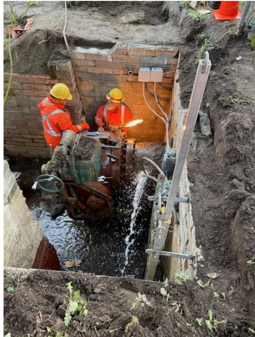
Removing 24-in ball valve
