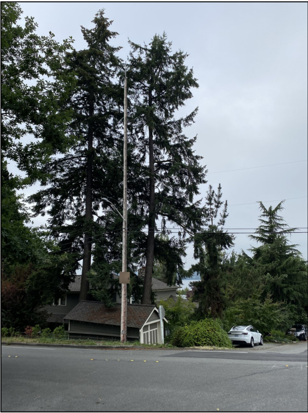
Photo rendering of example pole replacement at West Mercer Way and SE 32nd St with data collector equipment
