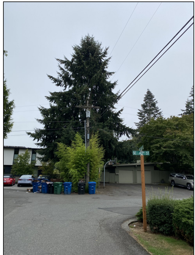
Photo of existing pole in Crestwood area (94th Ave SE & SE 43rd St)
