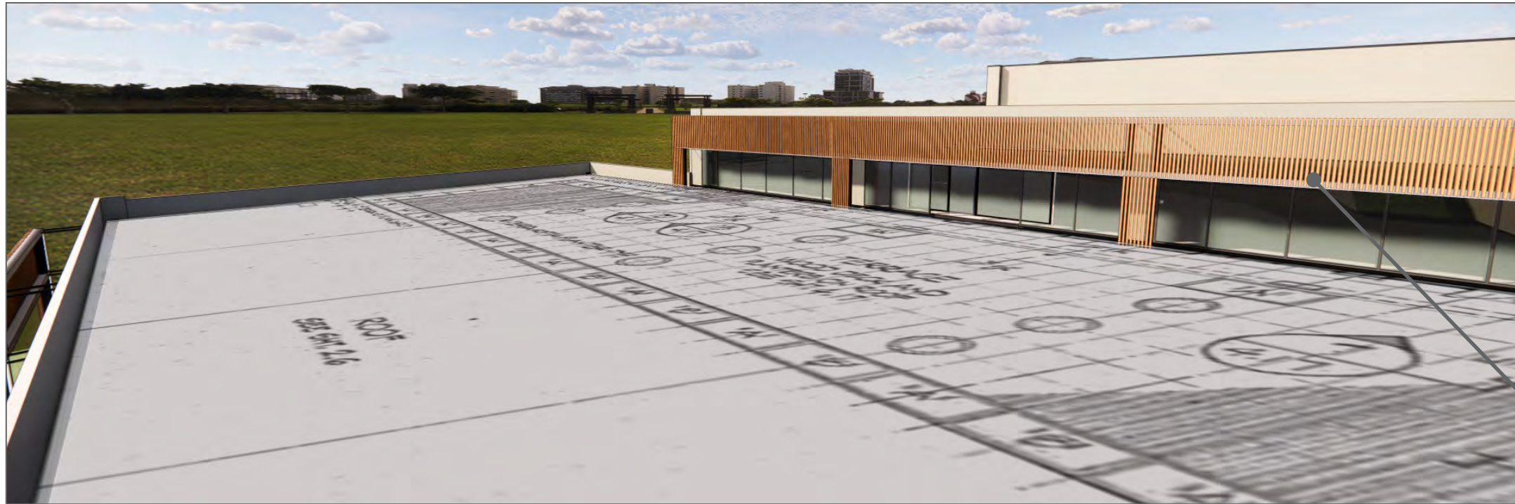
EXISTING SCREEN WALL TO BE REMOVED SO THAT A NEW UPDATED LOOK CAN BE PROVIDED.
