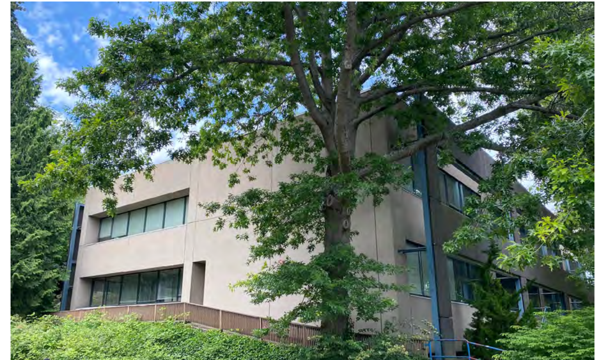
EXISTING THE EXISTING VIEW OF THE ROOF DECK. THE TREES HIDE MOST OF THE BUILDING.
