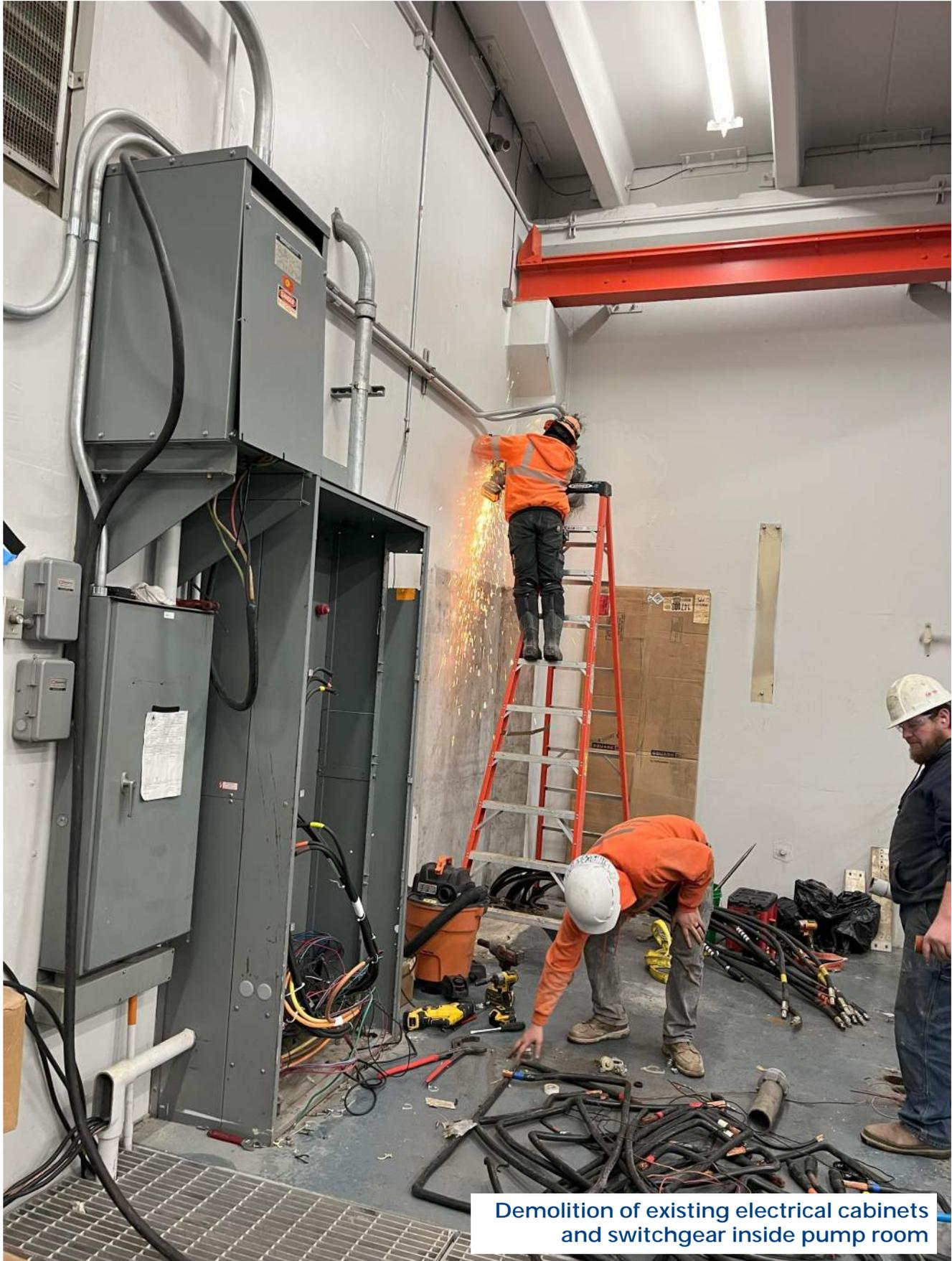
Demolition of existing electrical cabinets and switchgear inside pump room
