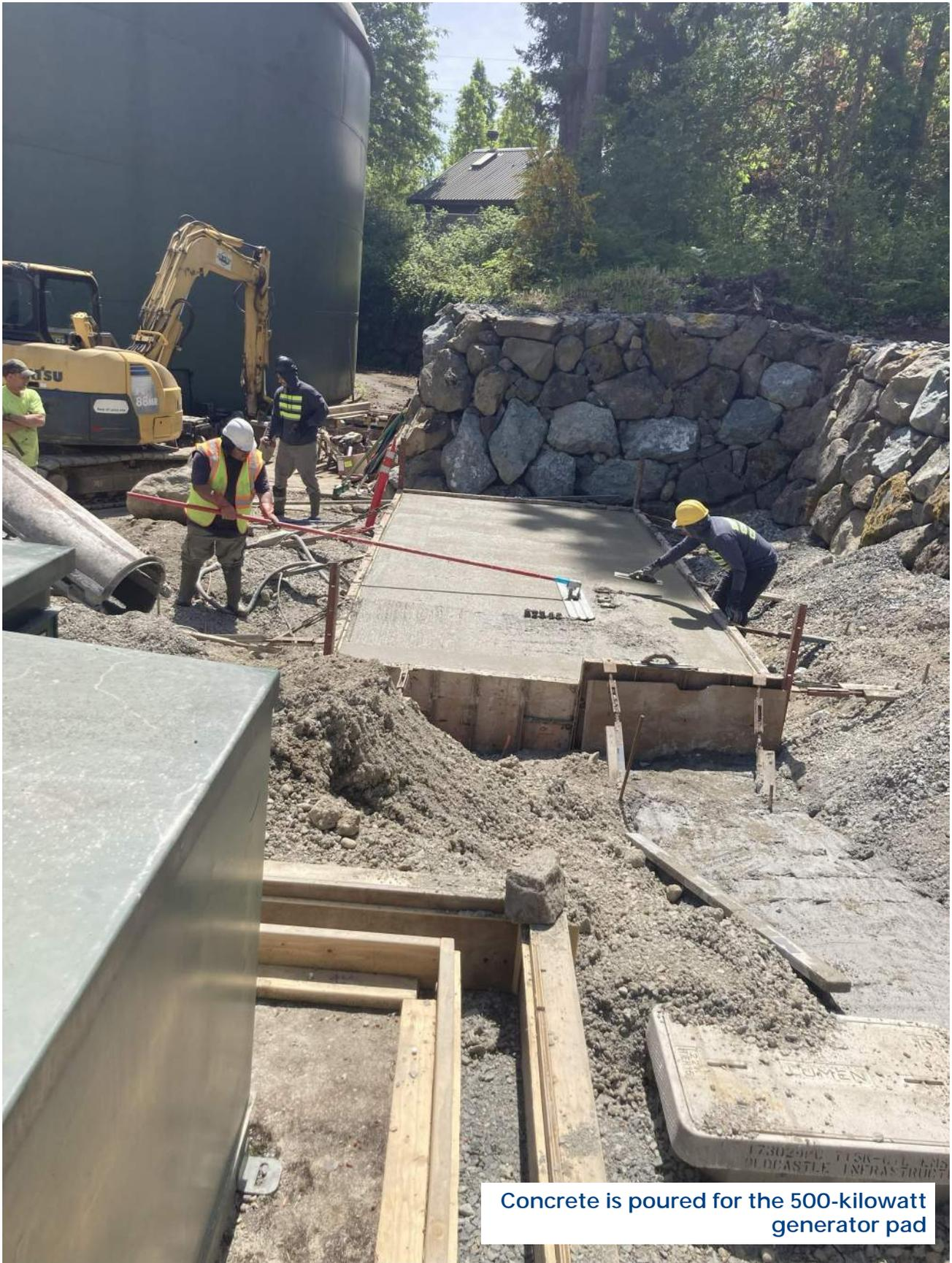
Concrete is poured for the 500-kilowatt generator pad
