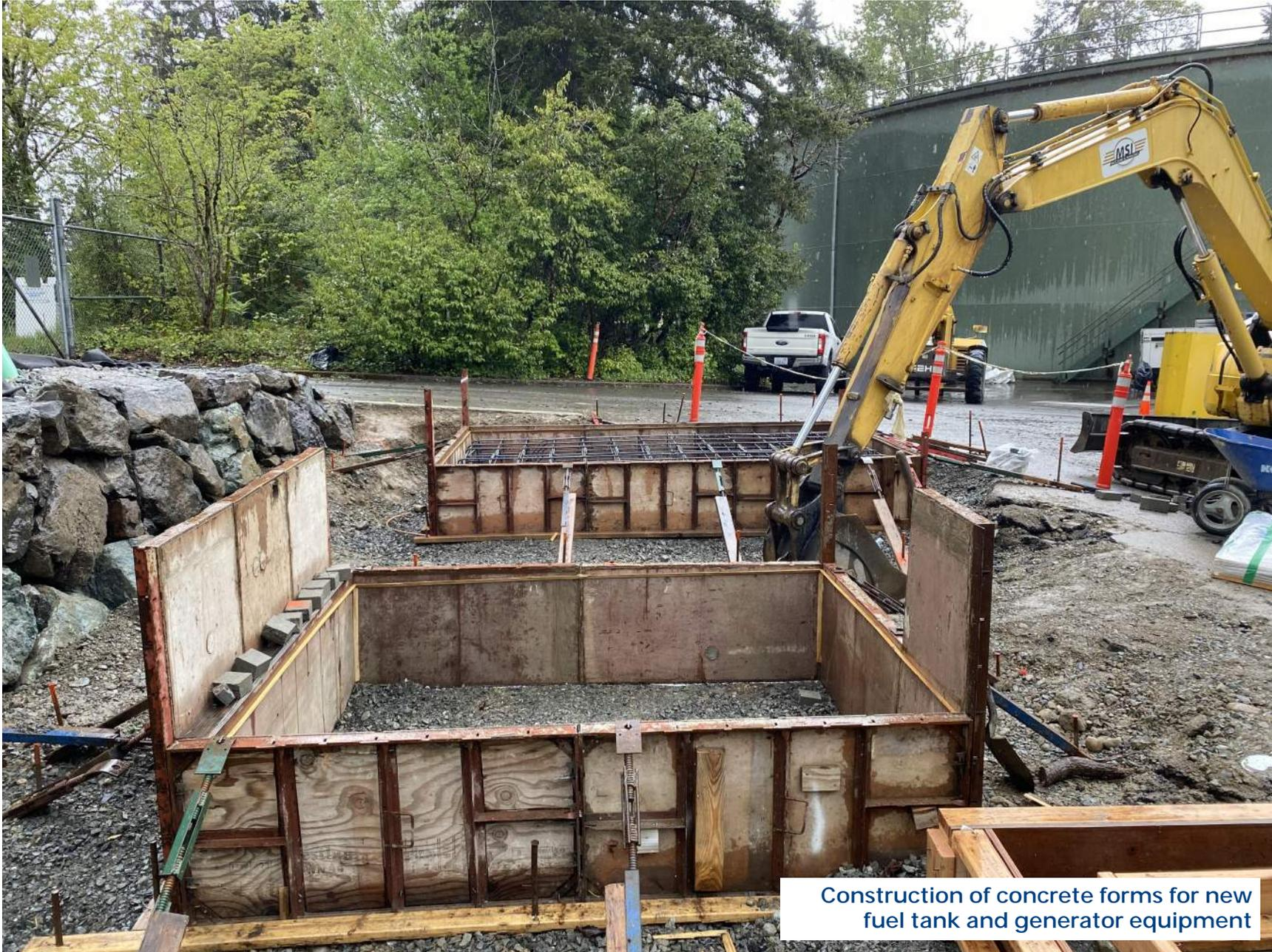
Construction of concrete forms for new fuel tank and generator equipment
