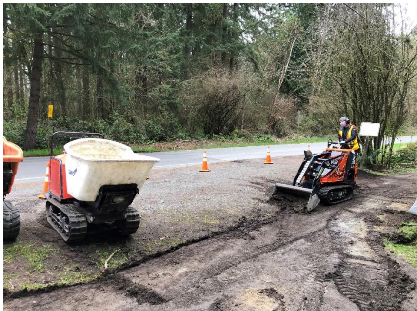
Natural Resources crew scraping away top surface
