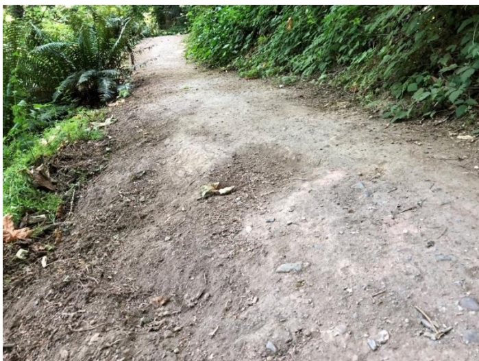
Trail surface eroding on steep sidehills
