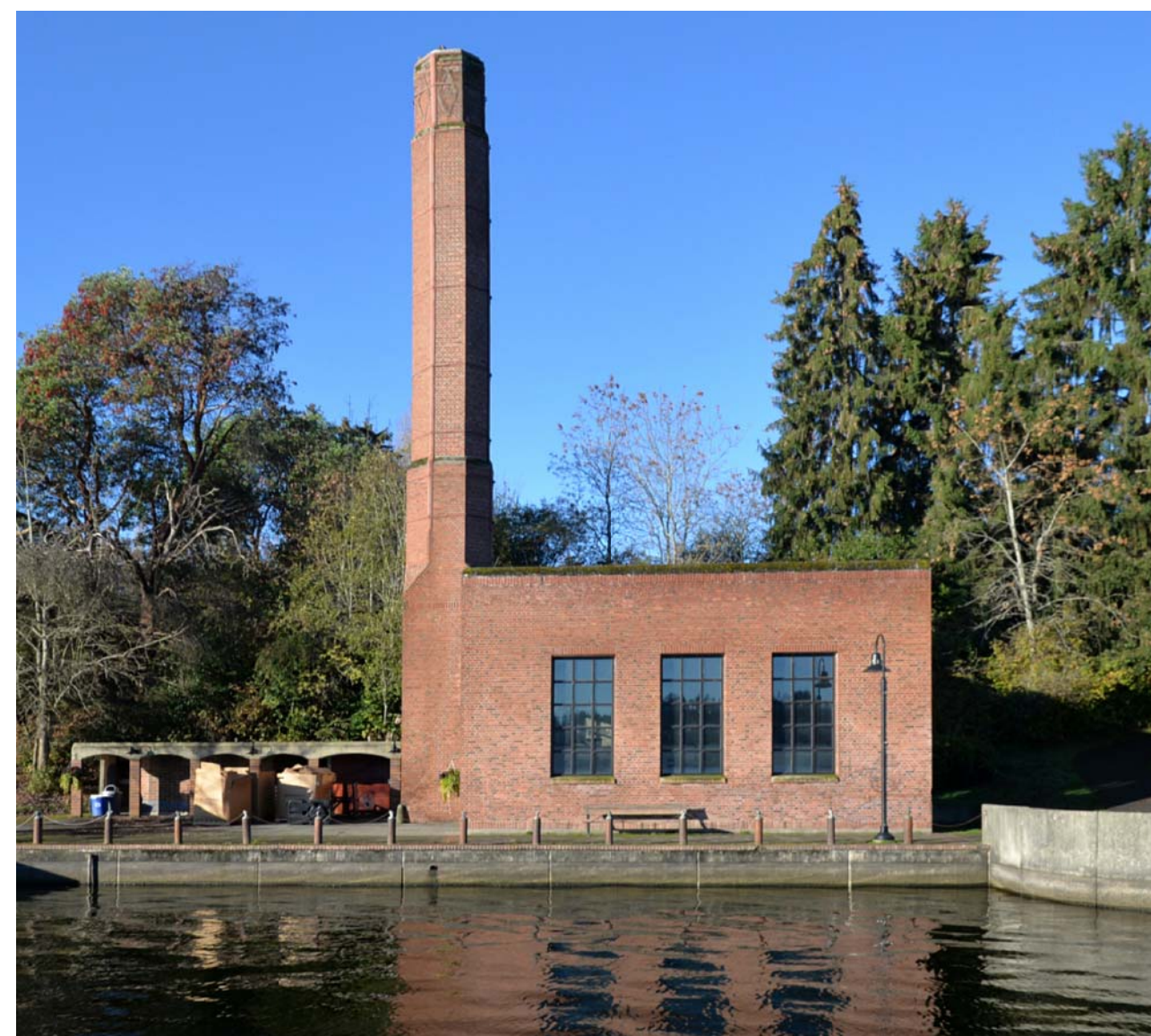
EXISTING BOILER BUILDING & STACK (2) NO SCALE
