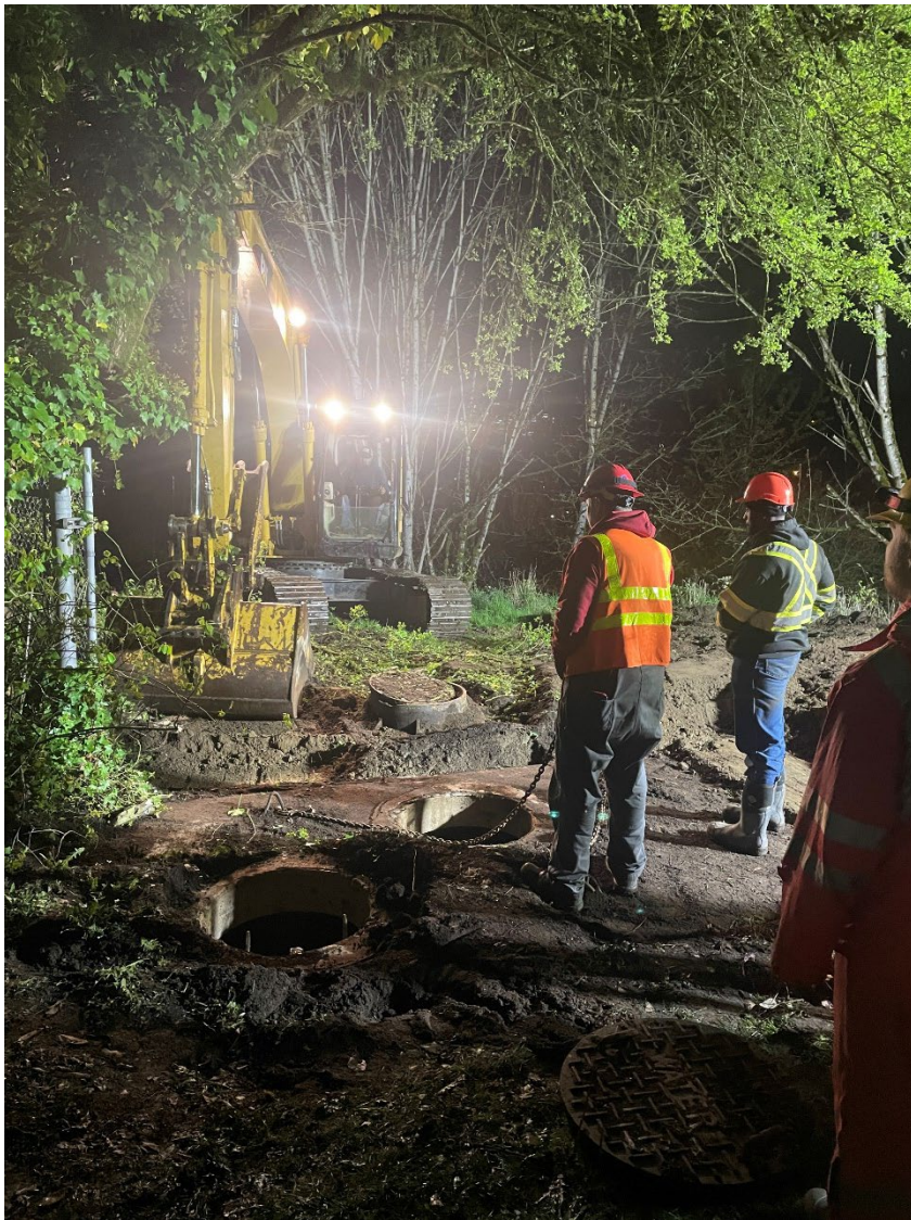
Valve vault before excavation
