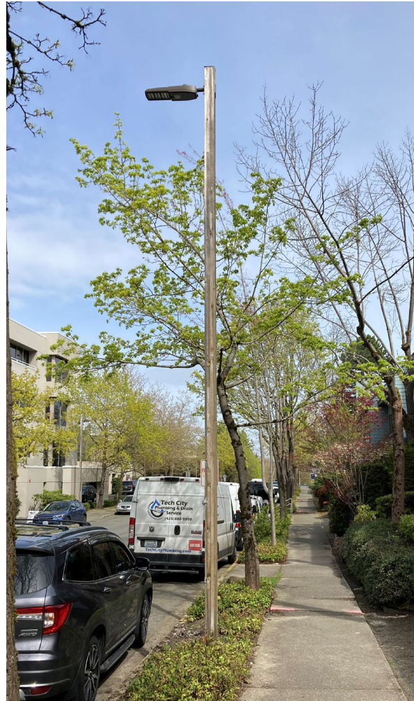
Typical wood pole to be replaced
