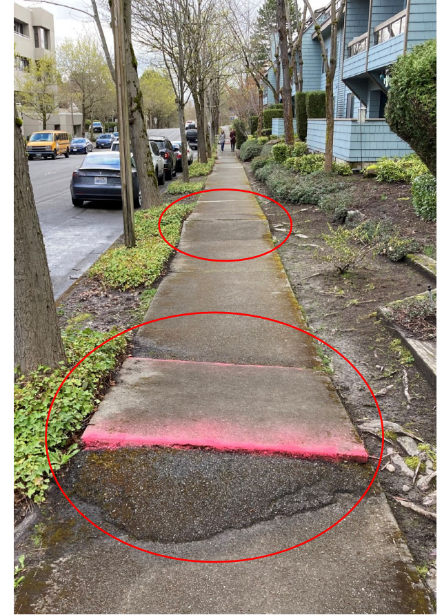
Does not meet ADA grade requirements
