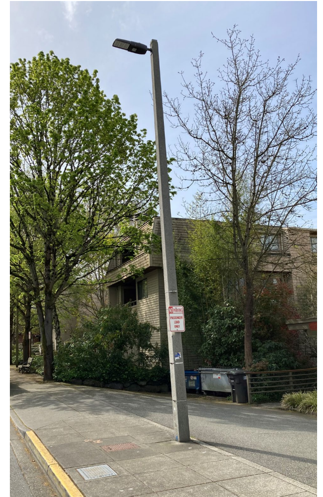
Typical concrete pole with LED light fixture
