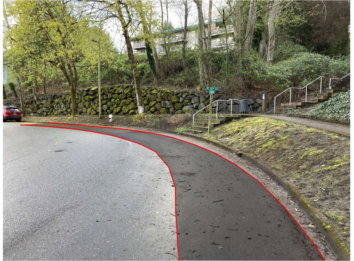
Grade difference between sidewalk and 80 th , new sidewalk to move onto street
