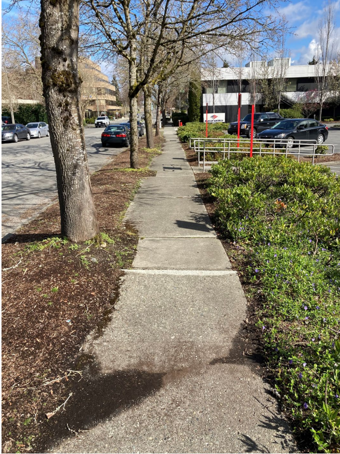
Raise grade of new sidewalk to save trees along Bank of America
