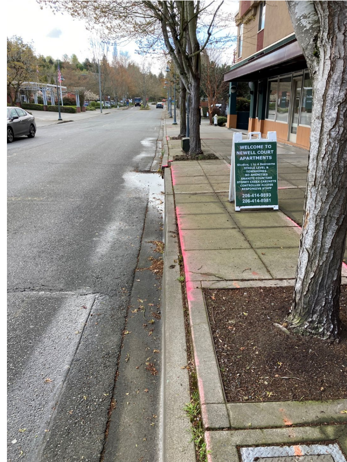
Curbs, sidewalks, and trees to be removed and replaced
