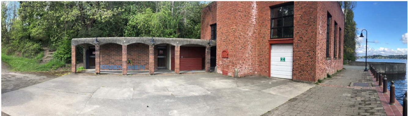
Figure 3: existing waterfront plaza with the boiler building on the right and restrooms on the left
