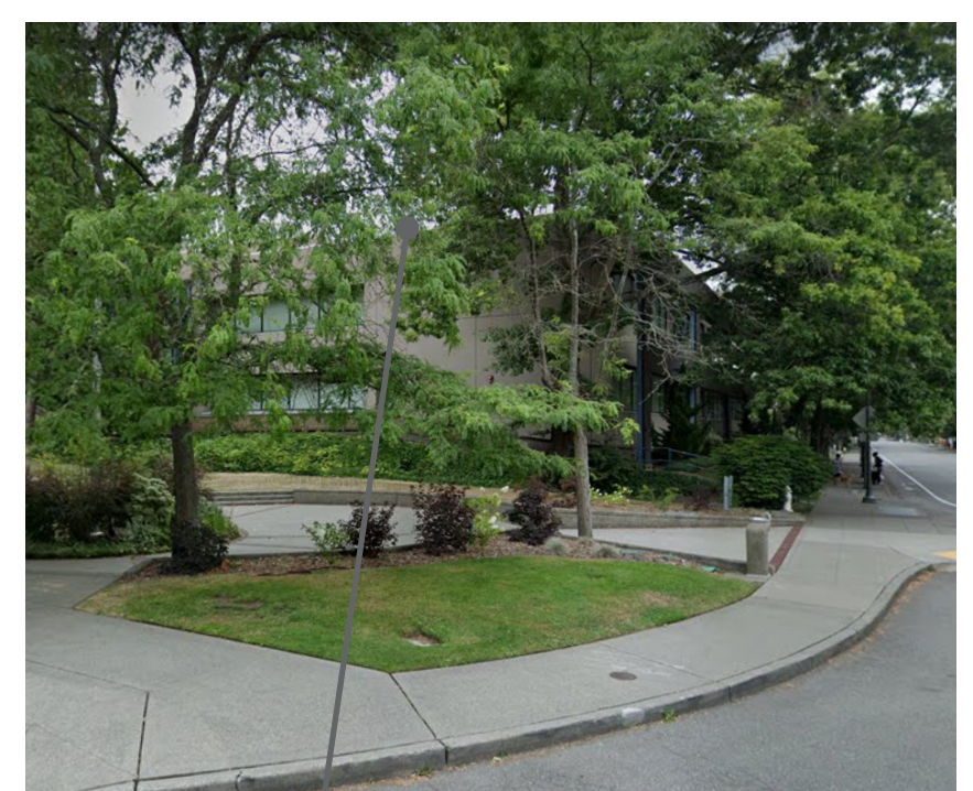
9 DOG HOUSE THIS EXTENSION OF THE EXISTING STAIR CASE TO THE ROOF TOP IS NOT VISIBLE FROM BELOW.
