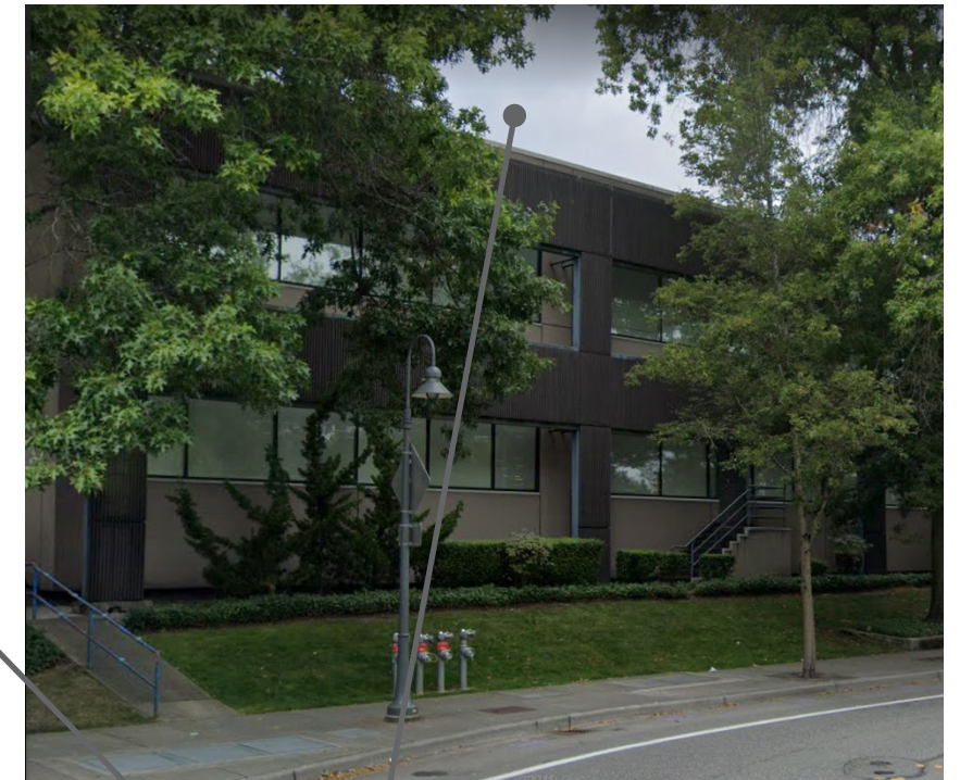
2 SCREEN WALL THE SCREEN AT THE FOURTH LEVEL DECK IS SET BACK ABOUT 70 FEET FROM EAST FACADE AND IS NOT READILY SEEN FROM STREET LEVEL.
