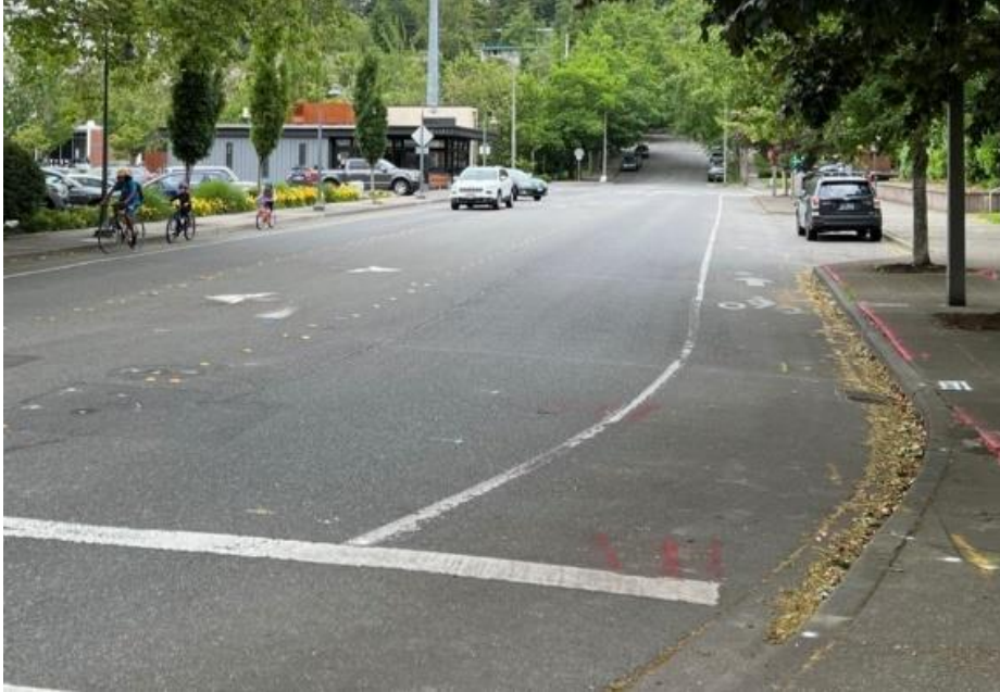
Image 15 Bike Lane Use on SE 32nd Street
