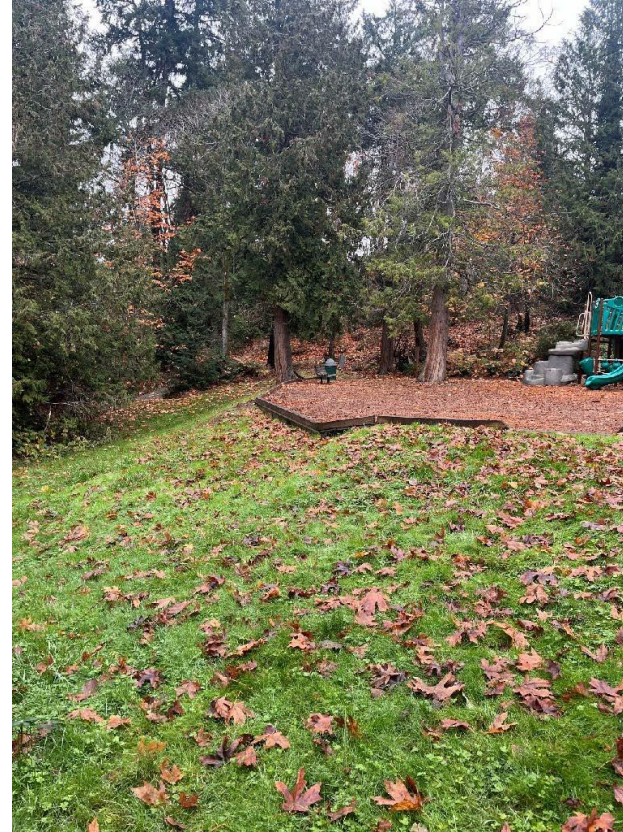
Surficial soil creep along the slope causes the western edge of the playground to settle.
