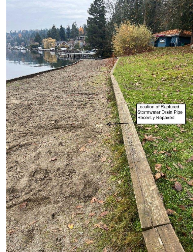
A stormwater pipe located in the beach area has been repaired twice after rupturing due to surface settlement.
