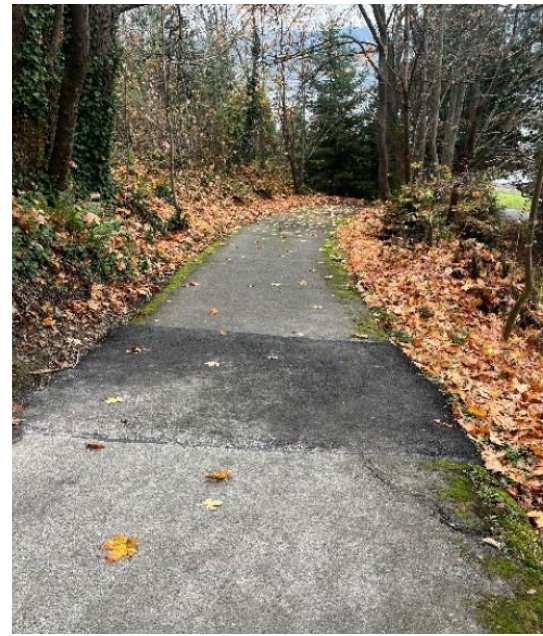
Soil creep throughout steep slopes causes asphalt cracking that must be routinely repaired.
