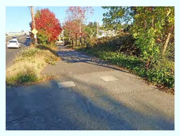
At locations where bollards are removed, the existing bollard and any in-pavement structural support should be removed in their entirety and replaced by a full repair patch. The repair patch should be a continuous surface with the surrounding trail surface.
