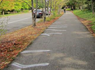
Trench along paving edge to stop tree roots from heaving adjacent paving. Install 18" depth root barrier to prevent future root problems.
