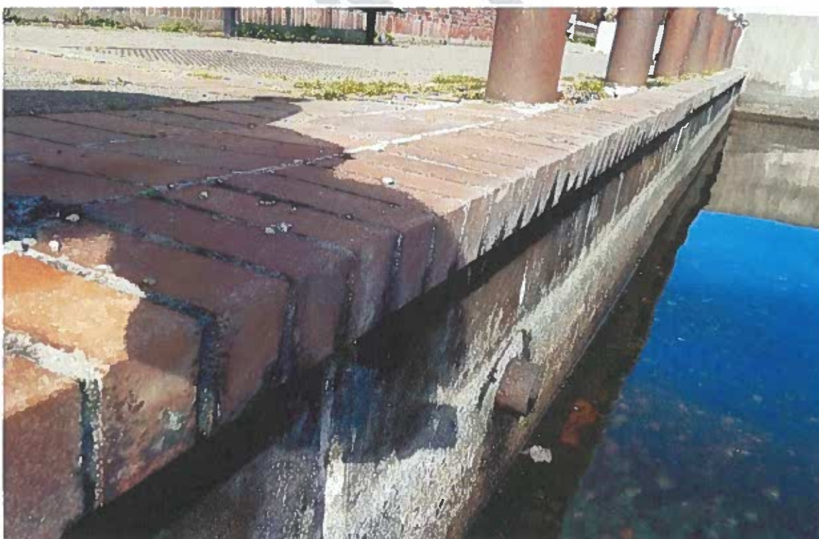
Figure 3. (B) One 4-inch diameter ductile iron pipe (2015).
