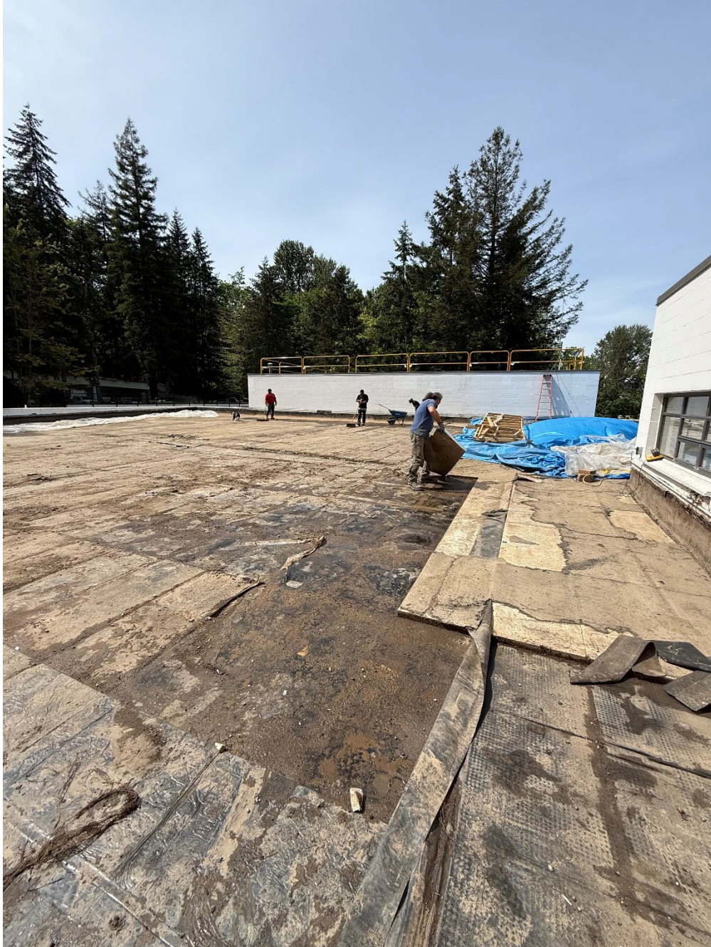
AB6901 | EXHIBIT 2 | GREEN ROOF ASSEMBLY REMOVAL
