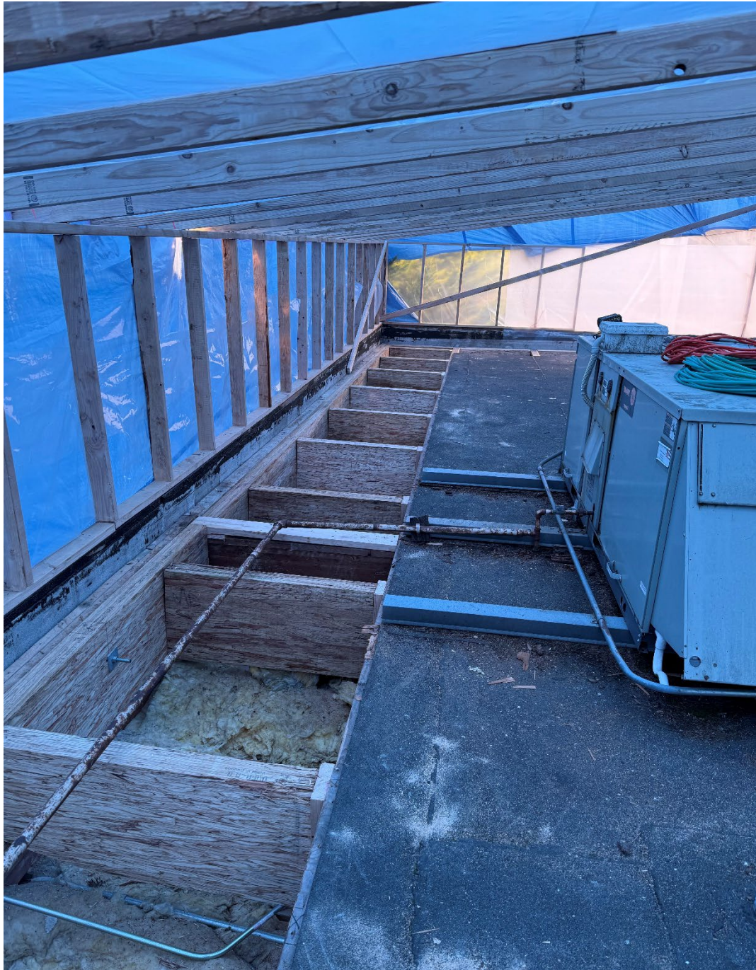
AB6901 | EXHIBIT 2 | UPPER ROOF REINFORCEMENT
