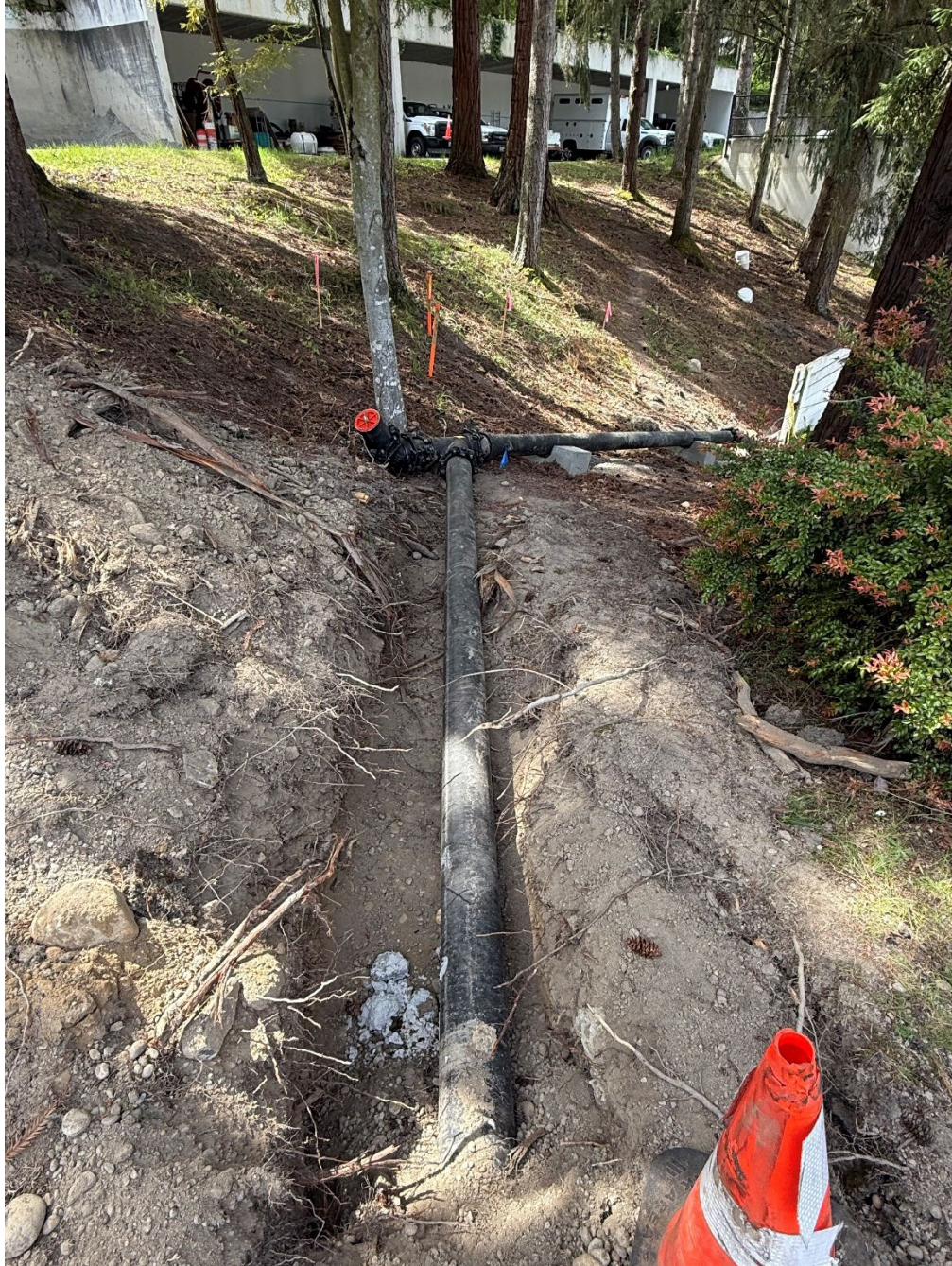
AB6901 | EXHIBIT 2 | STORM DRAINAGE INSTALLATION
