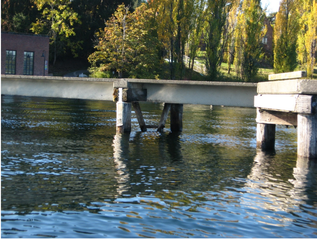
Figure 1: Profile view of pier showing concrete panel and wood cap beam construction
