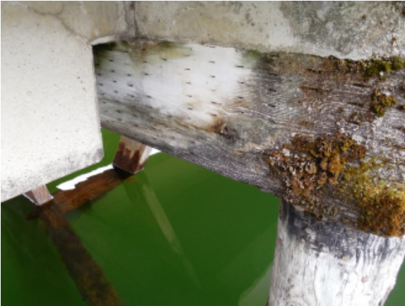
Photo 13A – Treated cap beam at pile
