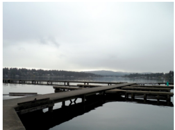
Photo 6A – Large pier
