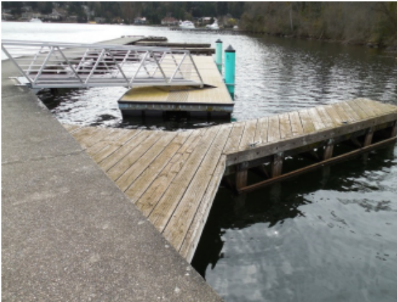
Photo 7A – Pier finger and gangway
