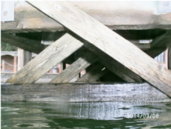
Photo 19A – Diagonal bracing
