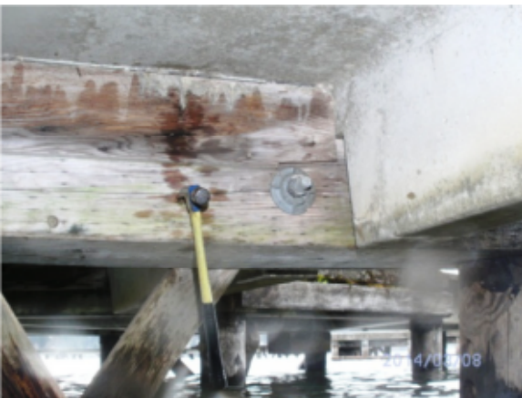
Photo 17A – Precast "T" and timber cap beam
