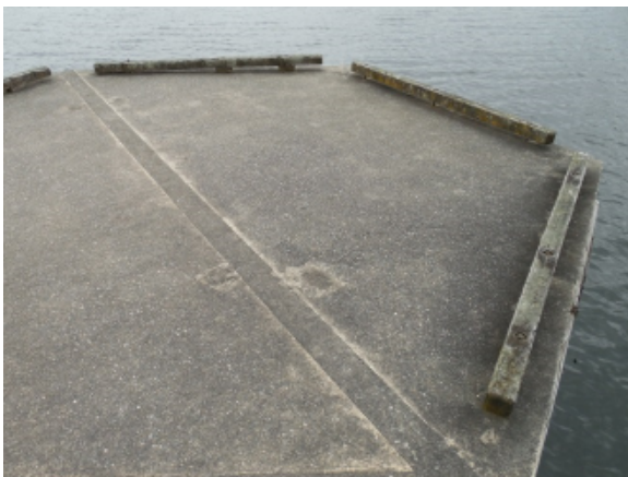
Photo 23A – Platform at end of small pier
