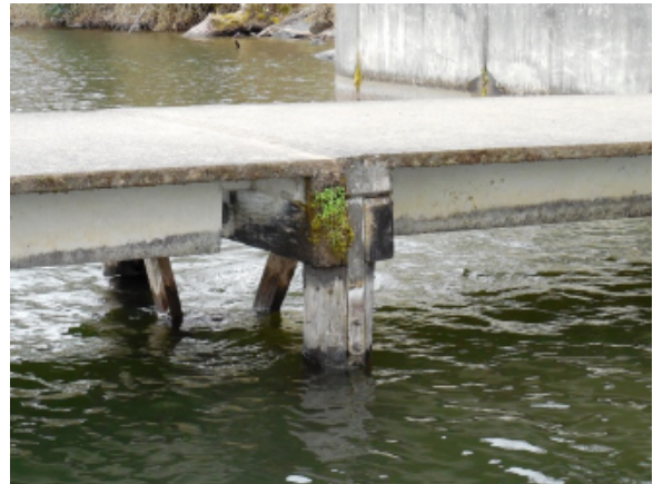
Photo 8A – Typical pier construction
