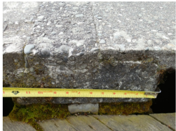
Photo 10A – Pier slab over support
