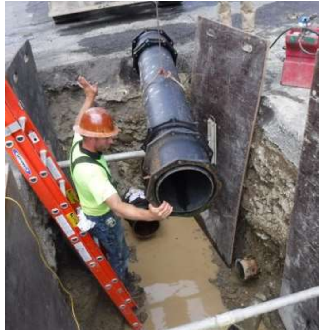
12" pipe installation
