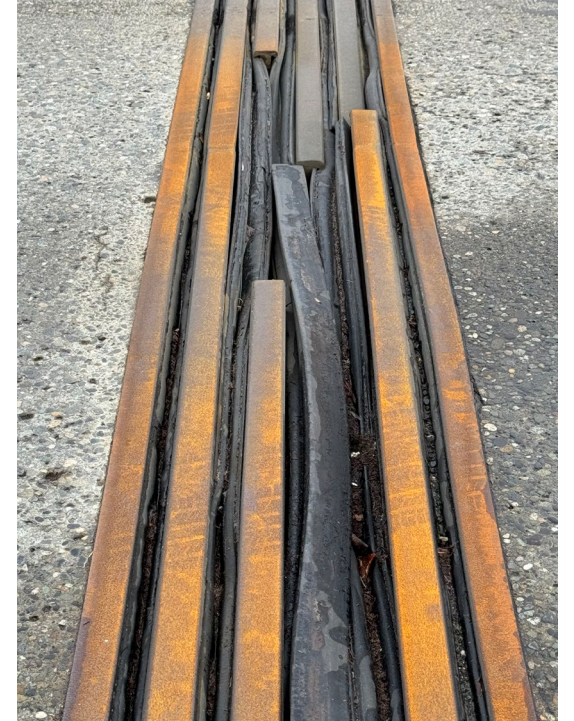
East Channel Bridge Failed Expansion Joint
