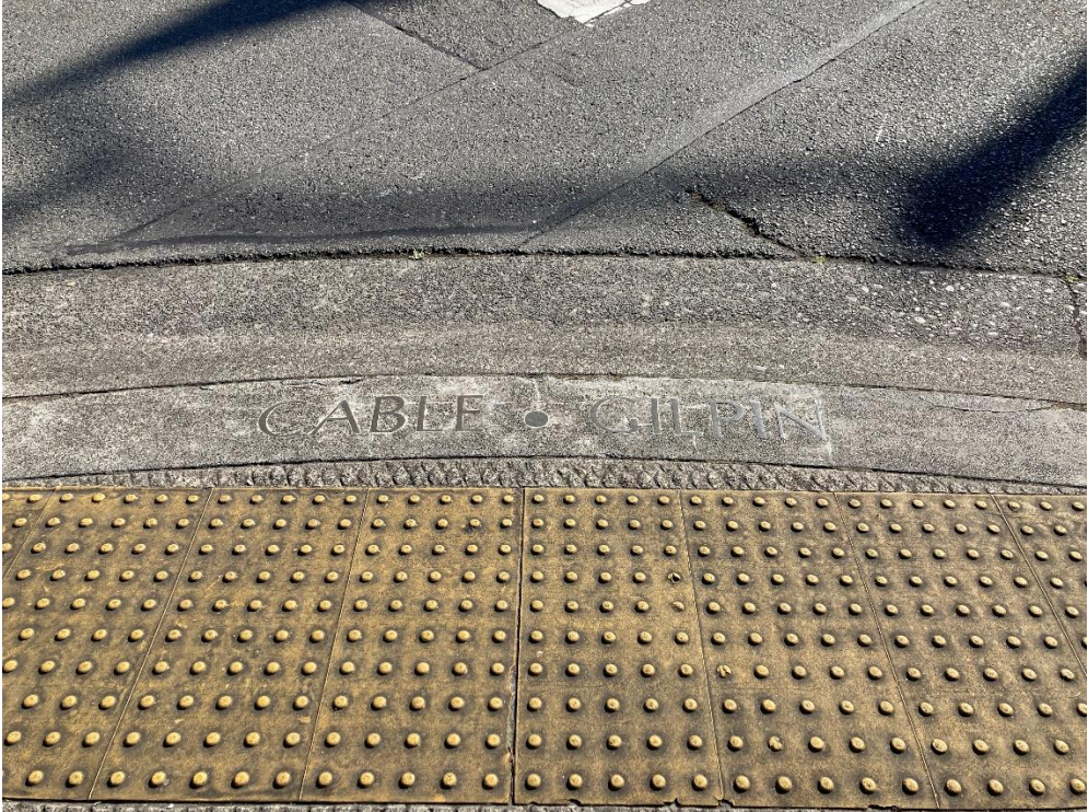
SW Corner: Cable-Gilpin
