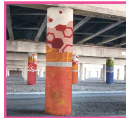
paint accent to overpass column $ +
