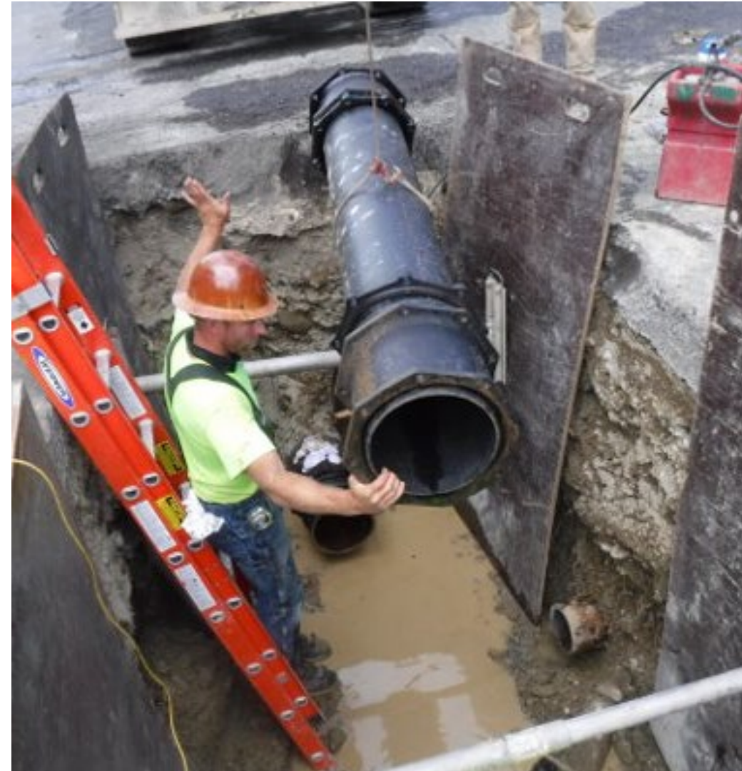
12" pipe installation
