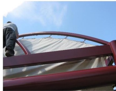
Hooks clip into welded "O" shaped rings on frame. There are approximately 30 clip areas.
