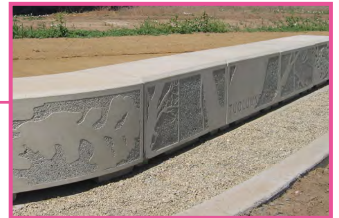
decorative sandblasted/etched seat walls example
