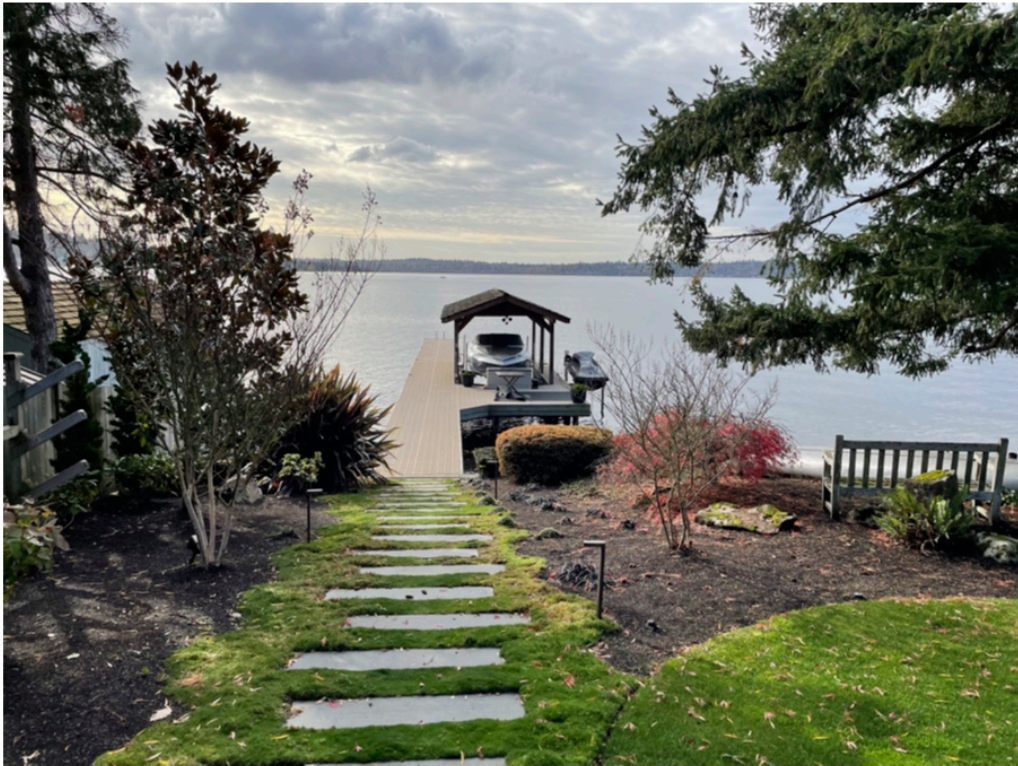
Photo 1 - Existing dock looking waterward.
