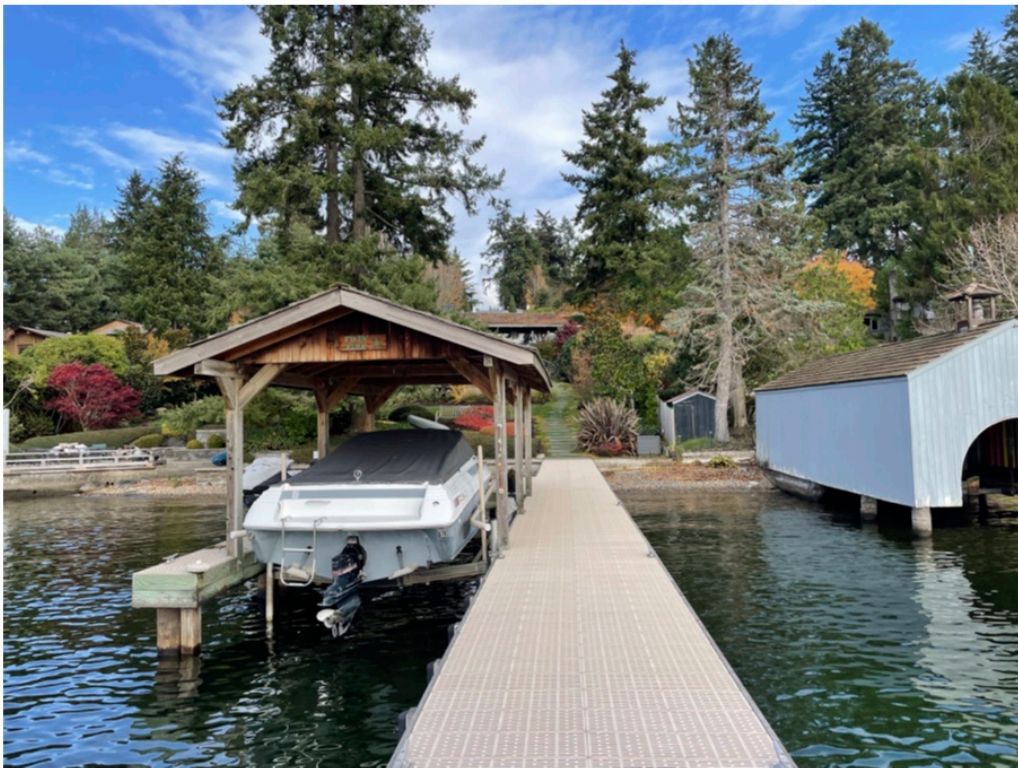
Photo 2 - Existing dock looking landward.
