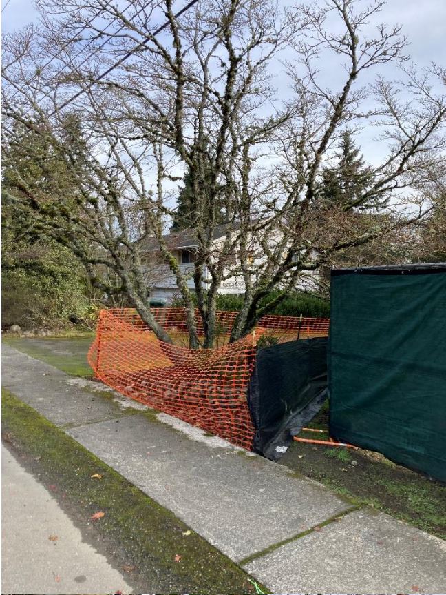
Picture 2. 2438 79th Ave NE – Tree protection inspection.
