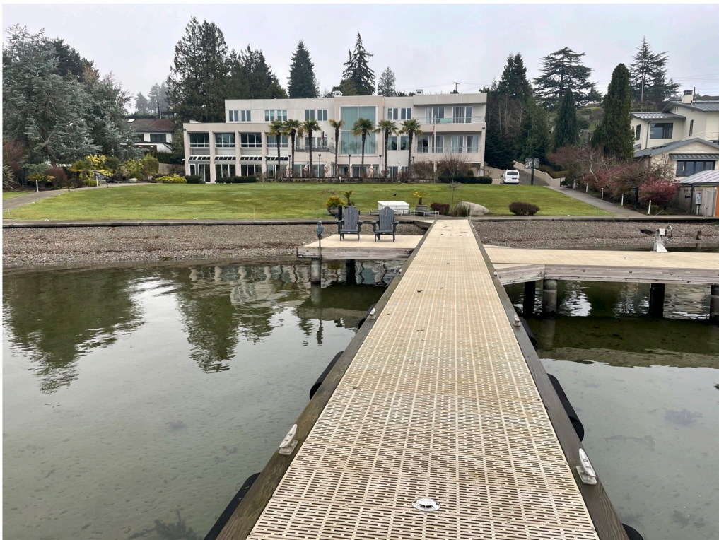
Photo 2 - Existing dock looking landward.
