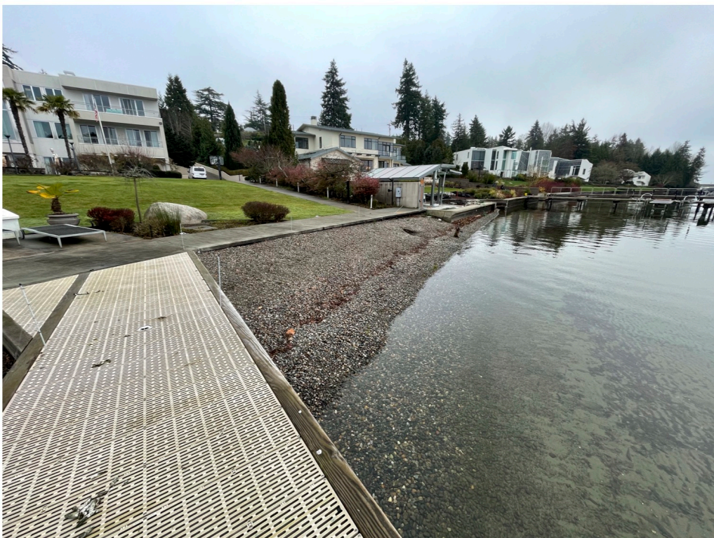
Photo 4 - Existing shoreline conditions looking south.
