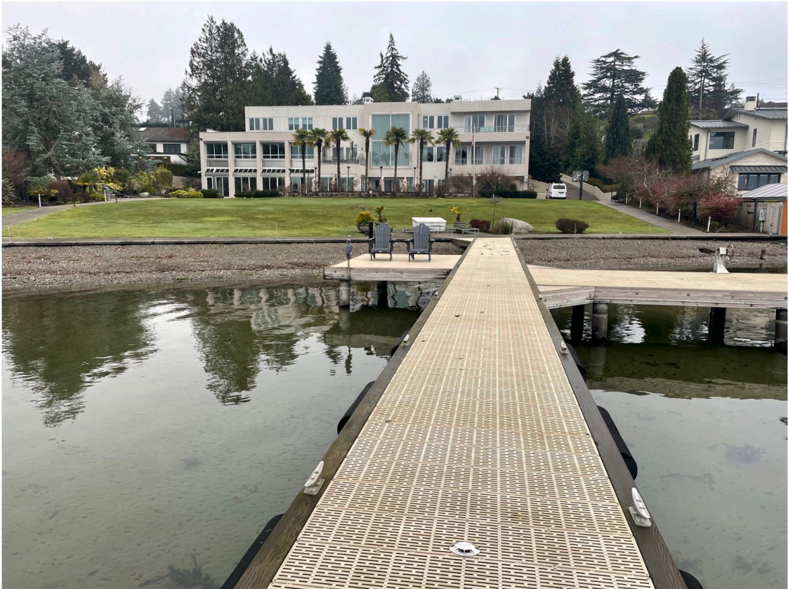
Photo 2 - Existing dock looking landward.
