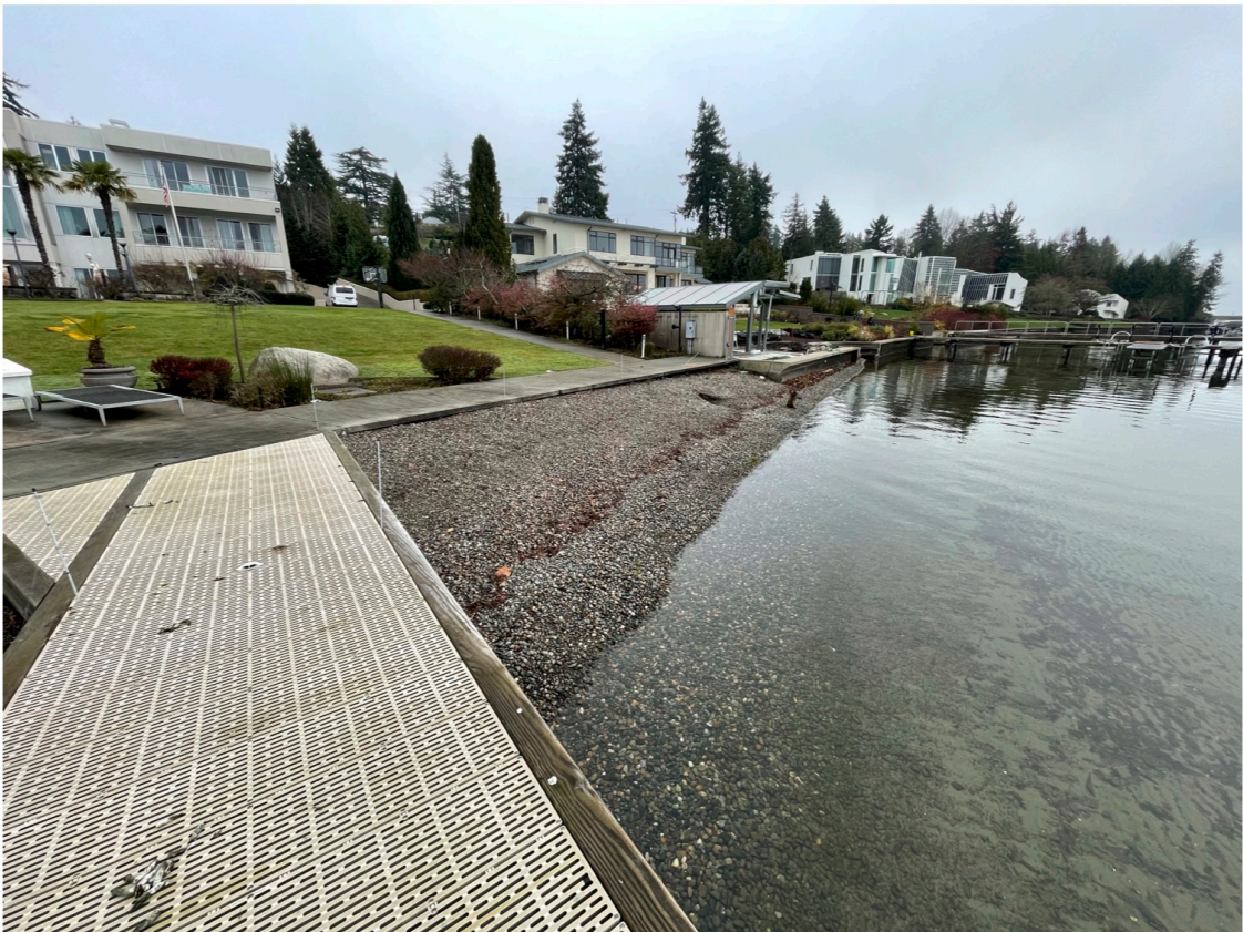
Photo 4 - Existing shoreline conditions looking south.
