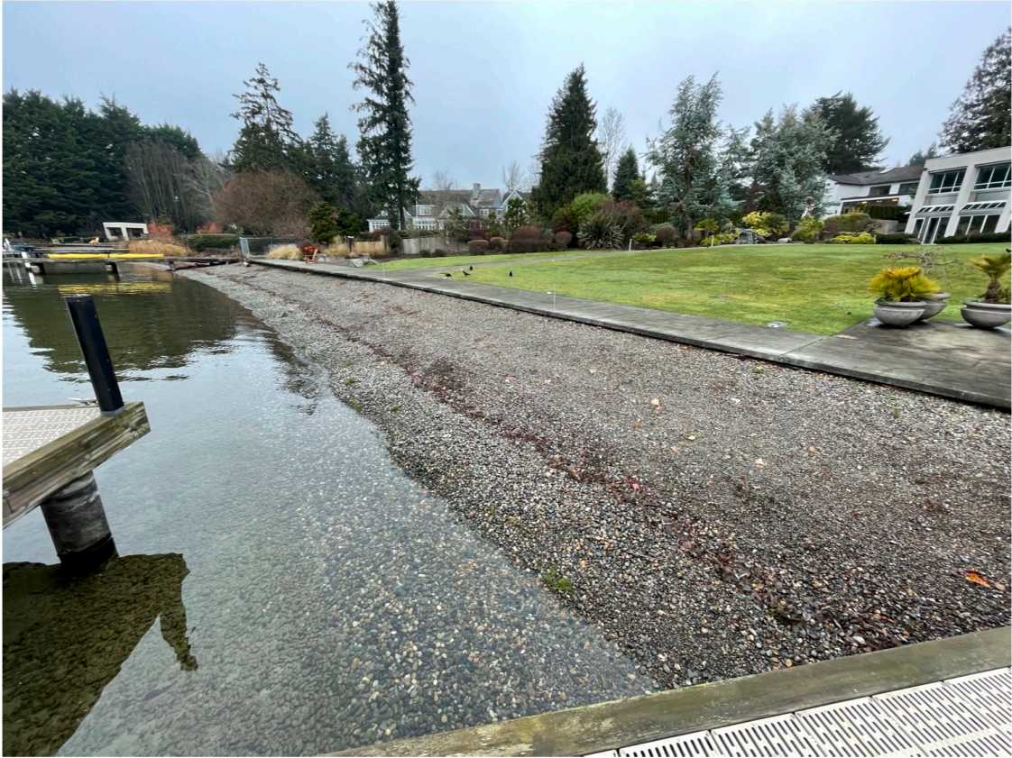
Photo 3 - Existing shoreline conditions looking north.
